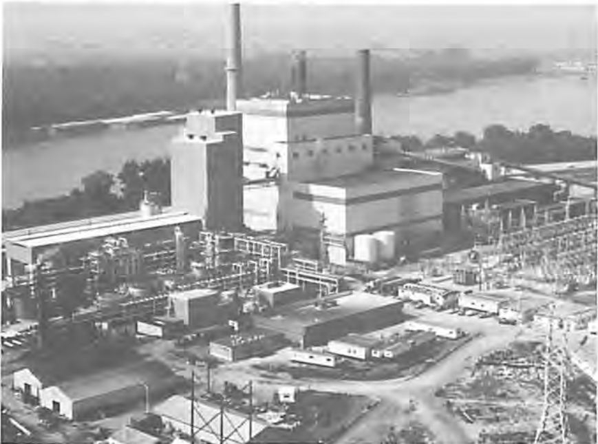
Fig. 2 – Aerial View of KILnGAS Commercial Module
