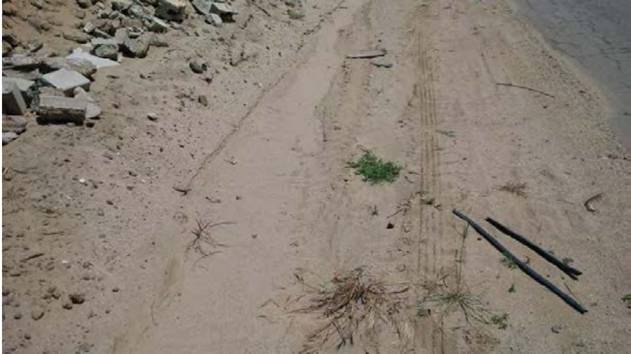
Photograph 7: Project: Bena Sanitary Landfill (SPK-2014-00236) Taken By: James Robb, USACE Date: May 8, 2014
