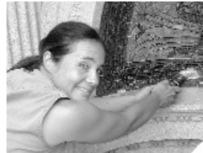
Art Preservation Technician Kimberly Carter removing old grout.
