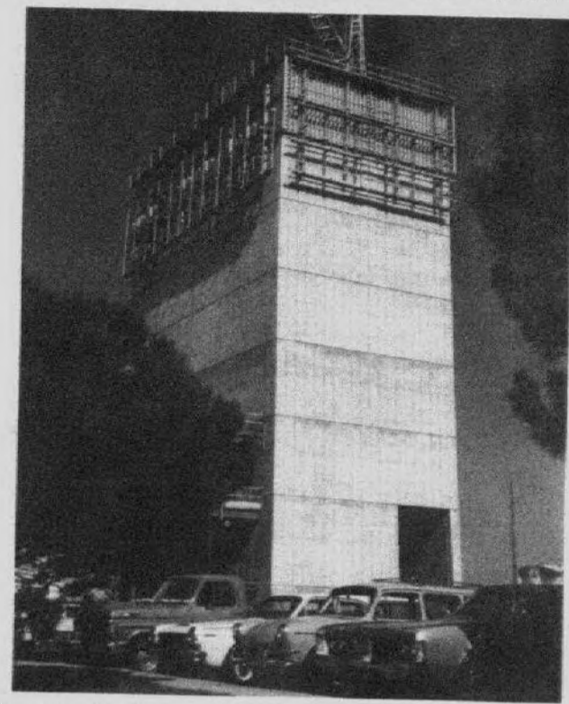
Newest addition to the skyline at NASA's Ames Research Center is this ten-story high structure which will house a new facility to simulate critical maneuvers of aircraft during take-off and landing. The new facility, called the Vertical Motion Simulator (VMS), will provide large up-and-down motions to simulate similar movement by aircraft such as the new Short Take-Off and Landing (STOL) and Vertical Take-Off and Landing (VTOL) vehicles of the future. Research pilots, riding in a simulator cab which can be configured to simulate various aircraft, will experience vertical excursions of up to 18 meters (60 feet) and 12 meters (40 feet) horizontally. The VMS is more advanced than any system now in existence and will for the first time have the ability to accurately simulate flare and touchdown of aircraft. Completion of the facility is scheduled in late 1976. The Carl N. Swenson Company of San Jose is constructing the building.
