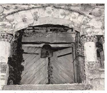
Scotsman's Island warehouse could transfer heavy guns through big doors directly to vessels for shipment.
