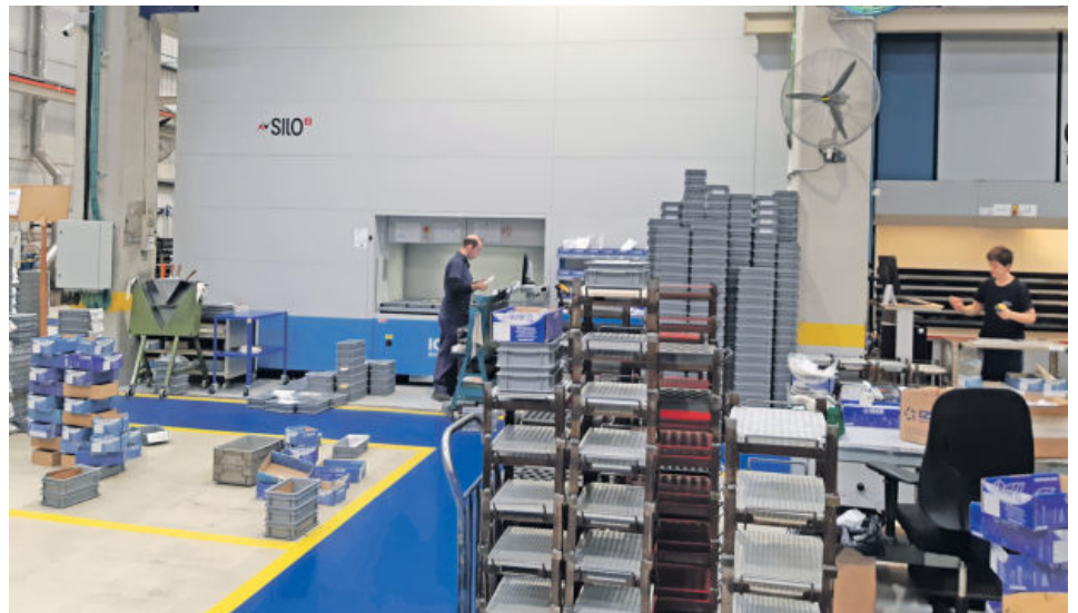
Its fourth automatic vertical warehouse will double its palletising capacity.
