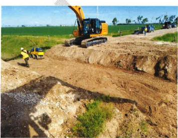
C. Last week we had a washout of a check on MC Canal. Had to dig out and rebuild. Still leaks. May have to rework in off-season.
