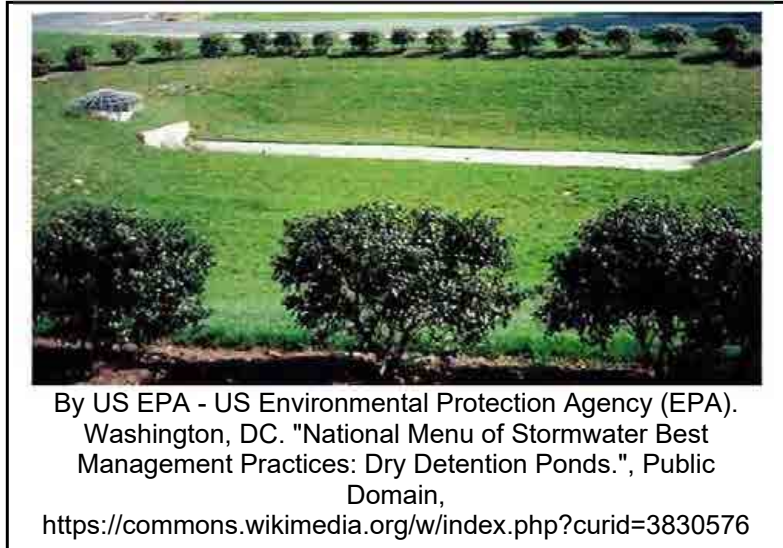
Figure 3-11 Example of a detention pond used for stormwater management from roadway runoff.
