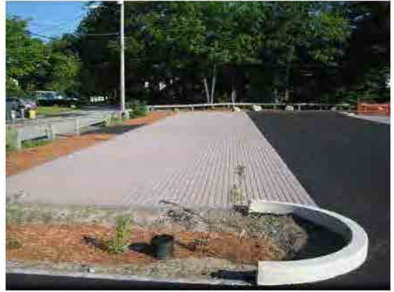
Typical green parking area with integrated planting areas and permeable pavers as per Massachusetts Executive Office of Energy and Environmental Affairs.
