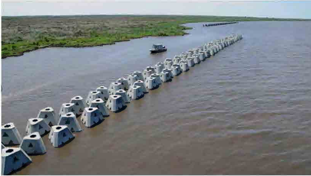
Figure 3-7 Wave attenuation devices 16
