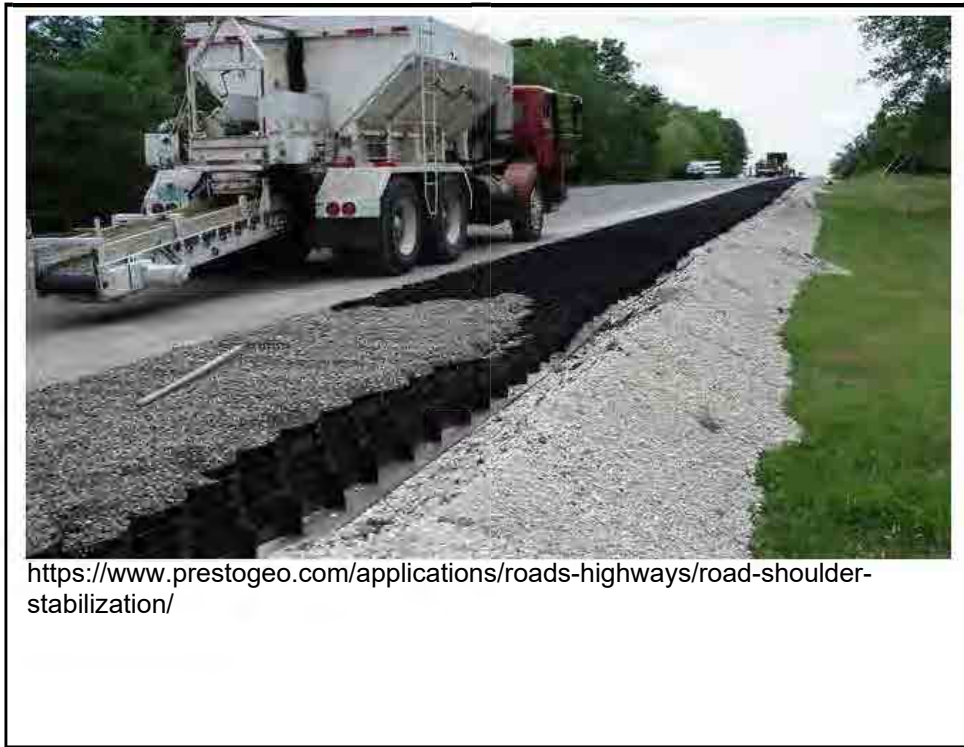
Figure 3-21 Installation of soil mats on a shoulder to reduce erosion and protect the road base against damage from water flow events.
