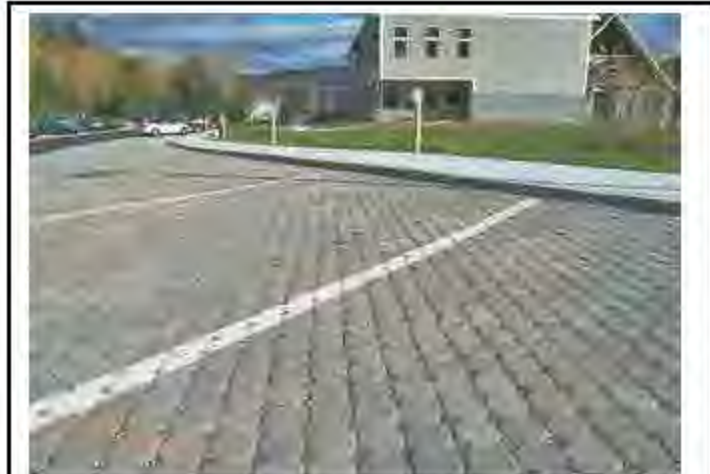
Figure 3-23 Installation of permeable pavers in a parking area to enhance drainage in a large space.
