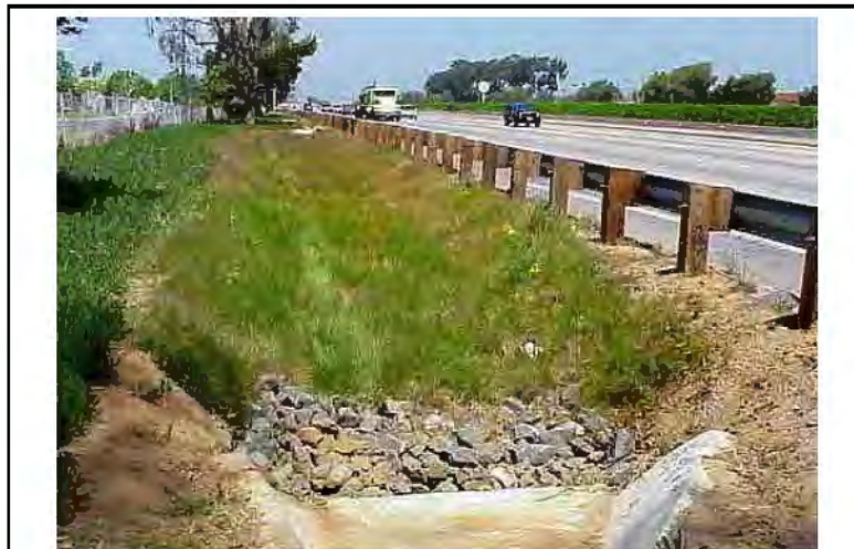
Figure 3-10 Example of a swale used for stormwater management from roadway runoff.
