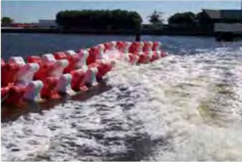
Figure 3-8 Floating wave attenuation device 17
