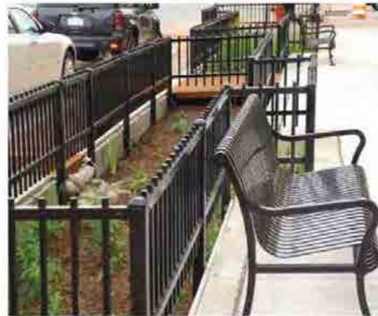
Michigan Avenue bioretention planter box Source: Tetra Tech, Inc.
