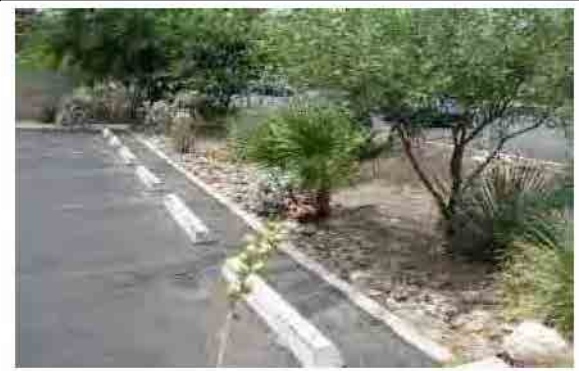
Typical green parking lot design as per EPA, "What is Green Infrastructure?"
