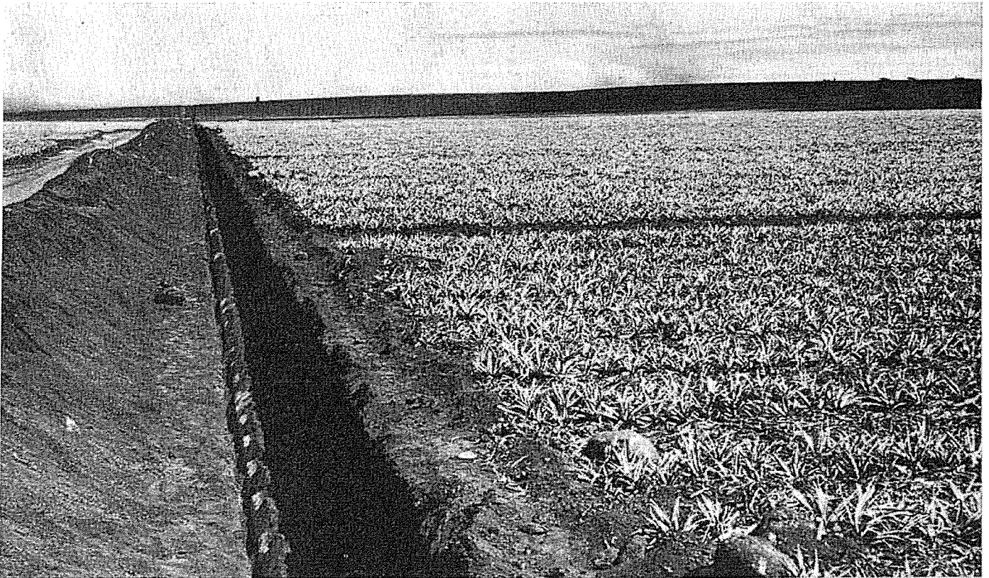
Figure 2.—An area of the Molokai-Lahaina association on Central Molokai showing part of Molokai Irrigation Project. Pipeline is buried at a depth of 6 feet. This association is used extensively for pineapple.
