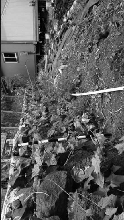
Figure 26: Photograph of Site -7552 Wall Three (3), View to North.
