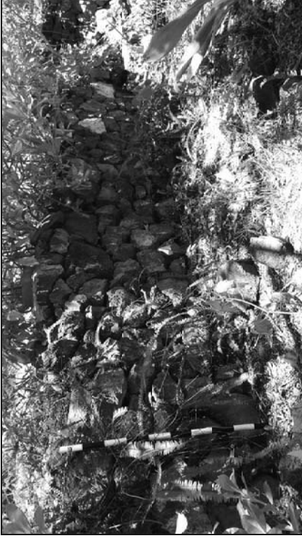
Figure 24: Photograph of Site -7552 Wall Two (2), View to North.
