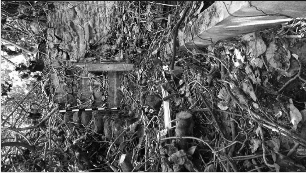
Figure 31: Photograph of Site -7553 Feature 1 (Wall with Attached Stairs). View to East.
