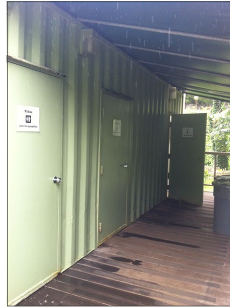
6. Restroom trailer to be replaced
