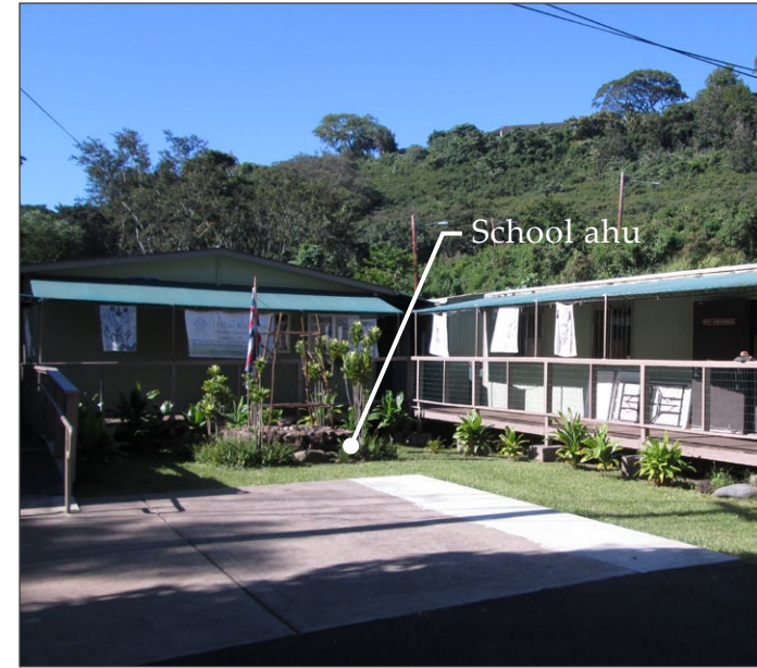
7. School ahu; Classroom trailer to be replaced (right)
