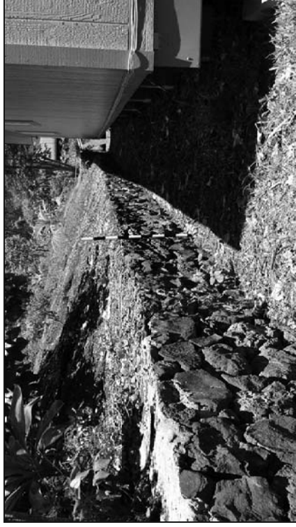
Figure 21: Photograph of Site -7552 Wall One (1). View to North.
