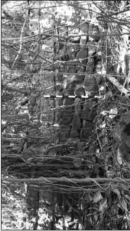
Figure 45: Photograph of Site -7554 (Stone Wall). View to East.
