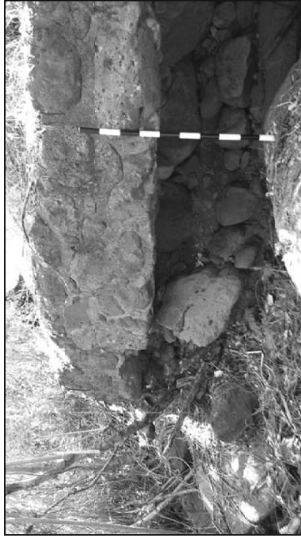
Figure 13: Photograph of Site -7550. View to West.
