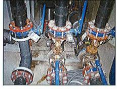
Removed Booster; Installed 4" Bypass
