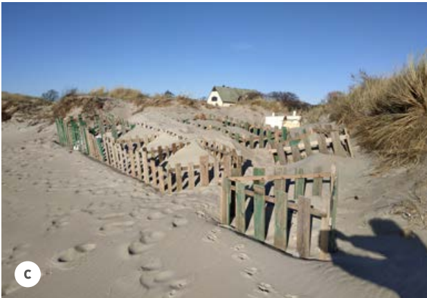
Figure 4.20. Experiment with wooden cells on the shore of the Vistula Spit: (a) the selected site (the right passage through the foredune), (b) construction process, December 2019, (c) after the wintertime, March 2020, (d) after the summer, with some grass already grown in triangular cells, which were preliminarily filled with beach wrack, October 2020. Photos: B. Chubarenko.
