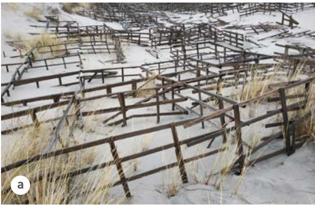
Figure 4.19. Beach wrack could be the best initial filler for wooden cells (a) used for sand accumulation, (b) in the wind-induced blowing gaps in the foredune wall, photos: B. Chubarenko.
