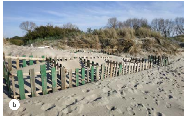
Figure 4.3. Experimental sites for beach wrack use for coast protection measures: (a) for greenery planting, (b) for sand accumulation constrictions, photos: (a) O. Rylkow, (b) B. Chubarenko.
