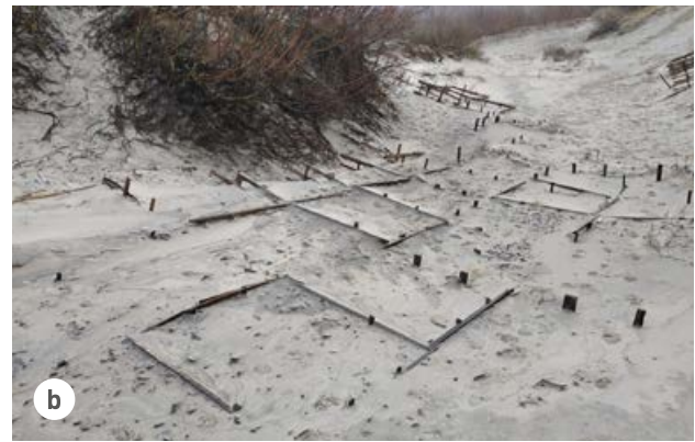
Figure 4.19. Beach wrack could be the best initial filler for wooden cells (a) used for sand accumulation, (b) in the wind-induced blowing gaps in the foredune wall, photos: B. Chubarenko.
