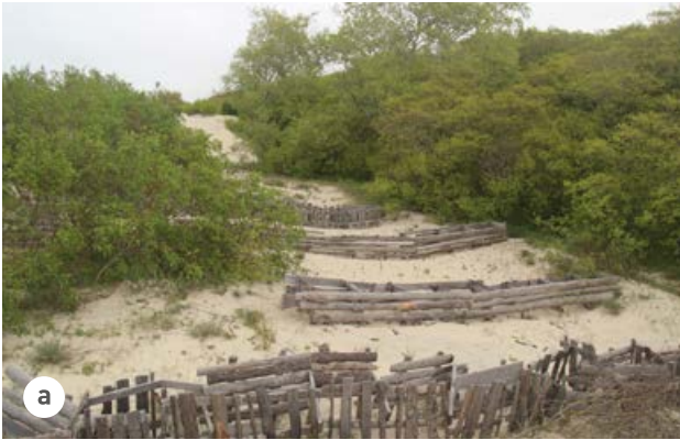
Figure 4.3. Experimental sites for beach wrack use for coast protection measures: (a) for greenery planting, (b) for sand accumulation constrictions, photos: (a) O. Rylkow, (b) B. Chubarenko.
