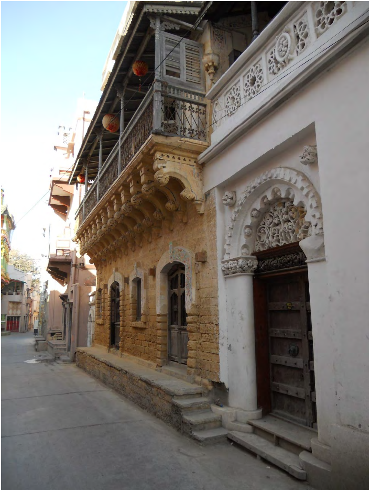
[Figure 4.12] Street view of urban house, Makata road, Diu, 2014.
