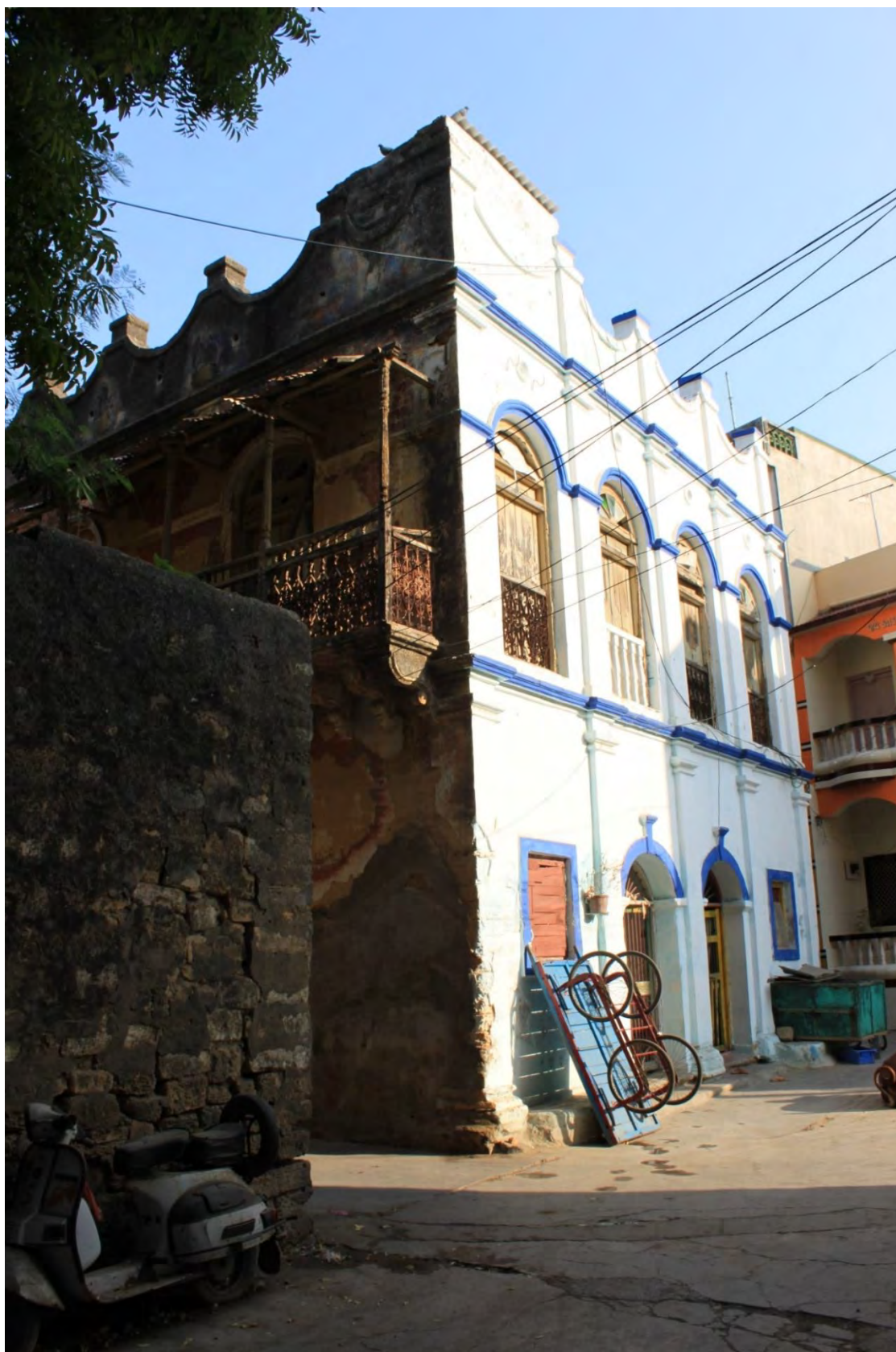
[Figure 4.17] Parsi house, Parsiwada , Diu, 2014.
