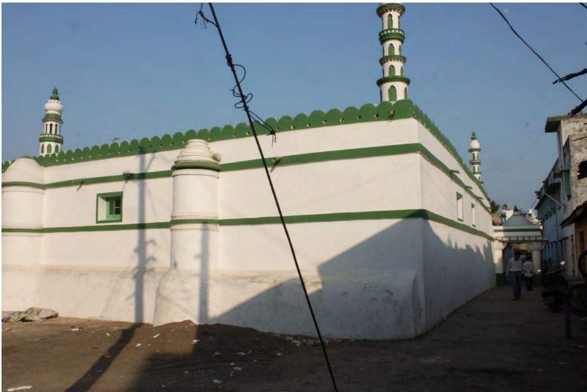
[Figure 5.17] Jami Masjid (main mosque) of Diu. Qiblah wall, west façade. 2014.
