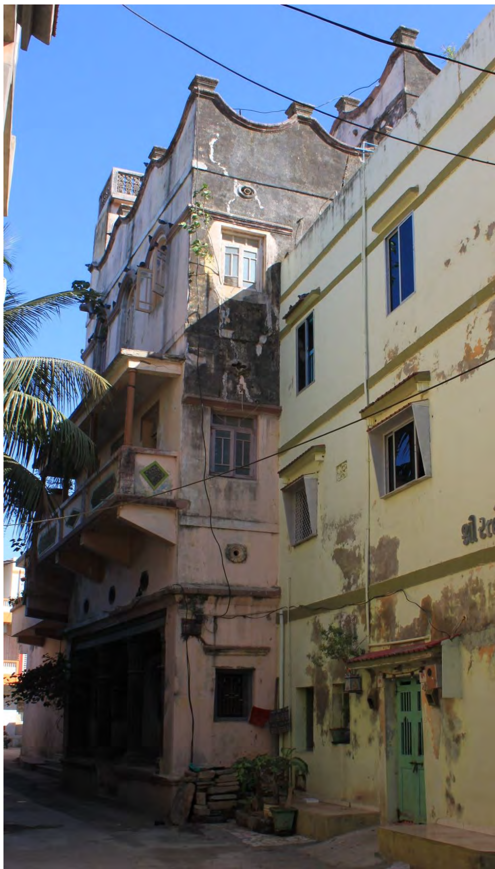
[Figure 4.16] Parsi house, Parsiwada , Diu, 2014.
