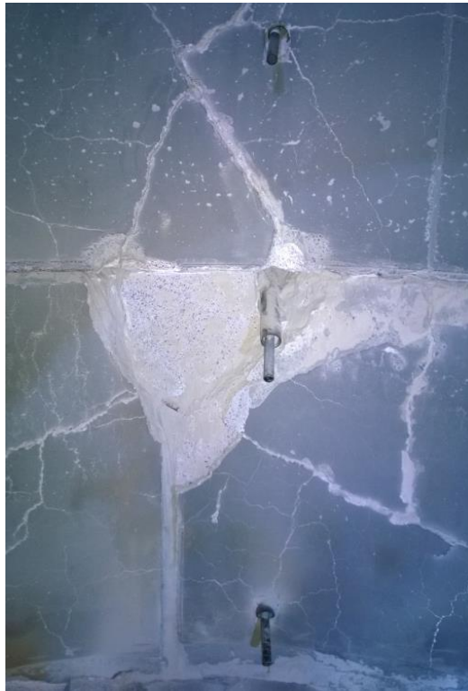
Figure 31: Refractory wall in CR (May 2014)
