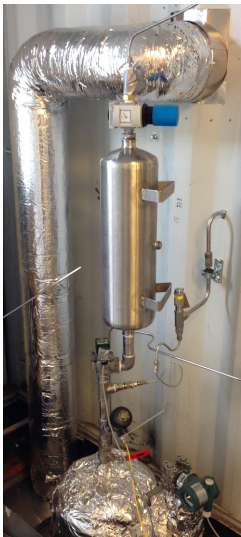
Figure 51: Filter blow back system
