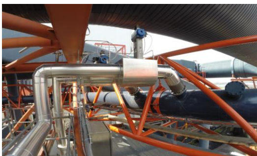
Figure 27: Pictures: Tar reformer installation
