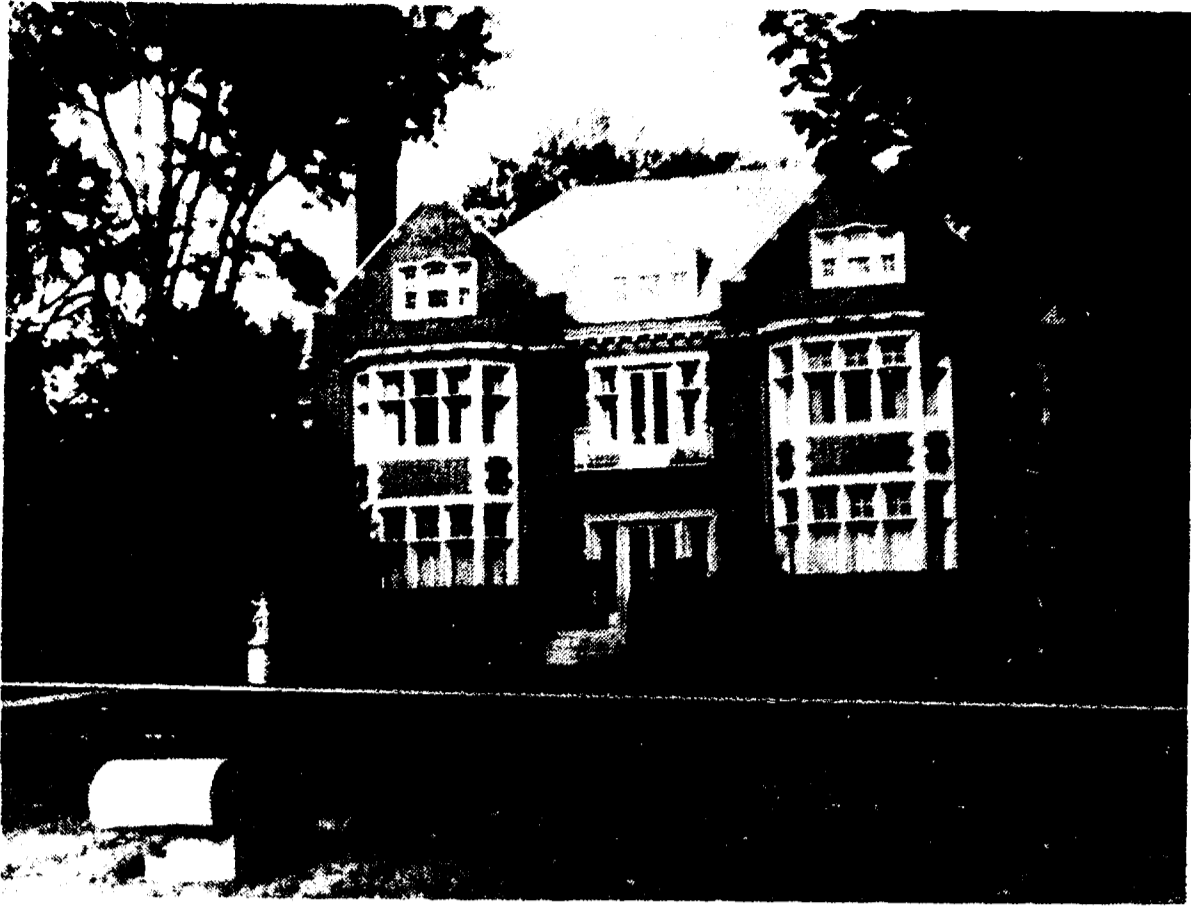
The Shelden Estate at 131 Lakeshore may be demolished early next year.
