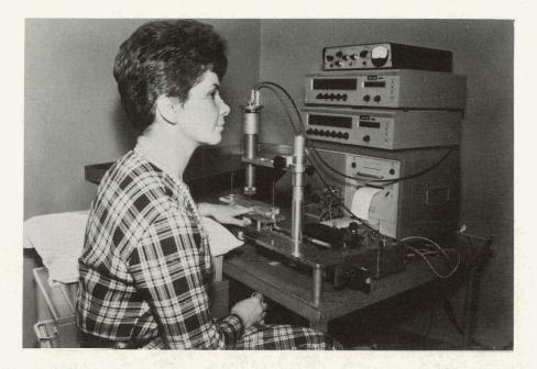
Figure 5. Subject with finger immobilized between plastic plates for counting. Data record appears on paper tape at lower right.
