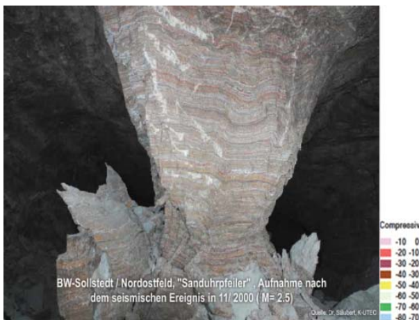
Figure 12 Hourglass pillar, Sollstedt mine, Northeast Field
