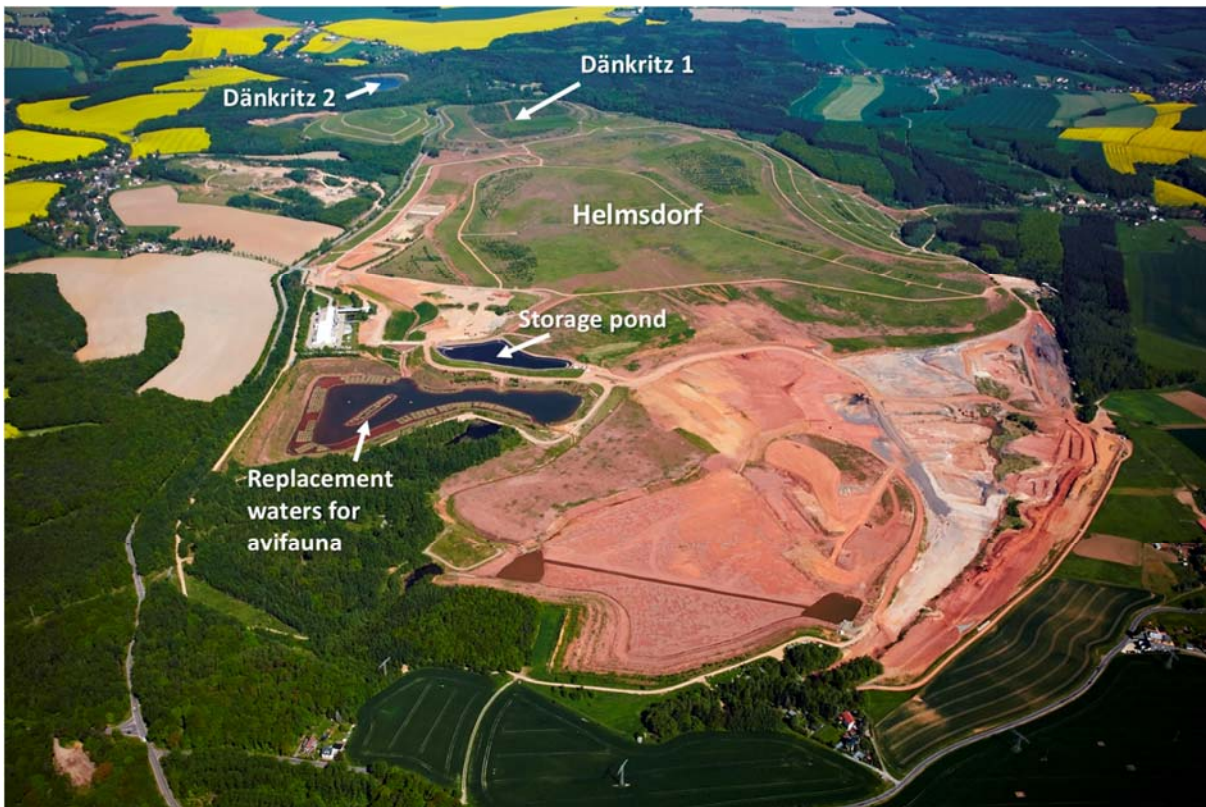
Figure 6 Aerial view of Helmsdorf/Dänkritz 1 TMF including replacement waters for avifauna (view from S to N, Oct. 2017)
