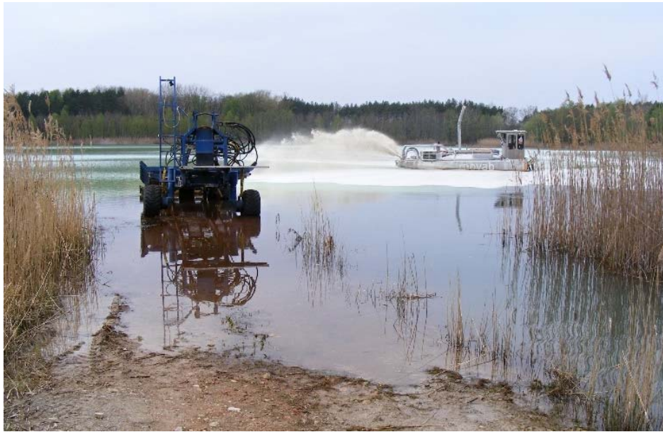
Figure 9 Mobile charging point at the lake Tröbitz, 2016
