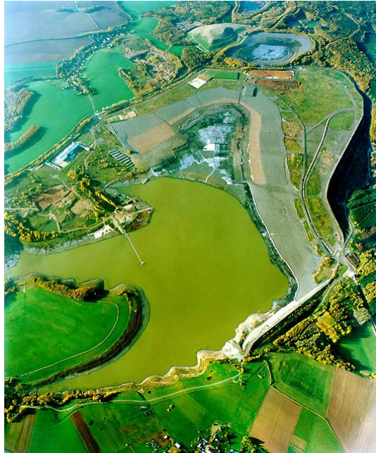
Figure 1 Tailings ponds Helmsdorf and Dänkritz 1 (background) in 2000 (WISMUT air photo L972/10)
