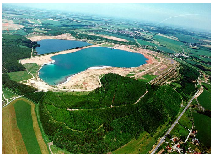
Figure 3 Tailings pond Culmitzsch in 1993 (WISMUT air photo: L 179/12)
