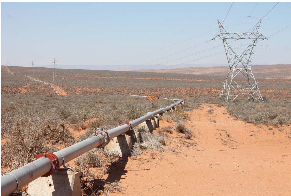
Figure 4 Drinking water is delivered to Kleinzee over a distance of 85 kilometres via a privately owned and operated pipeline. The electricity distribution and reticulation infrastructure is also privately owned and operated
