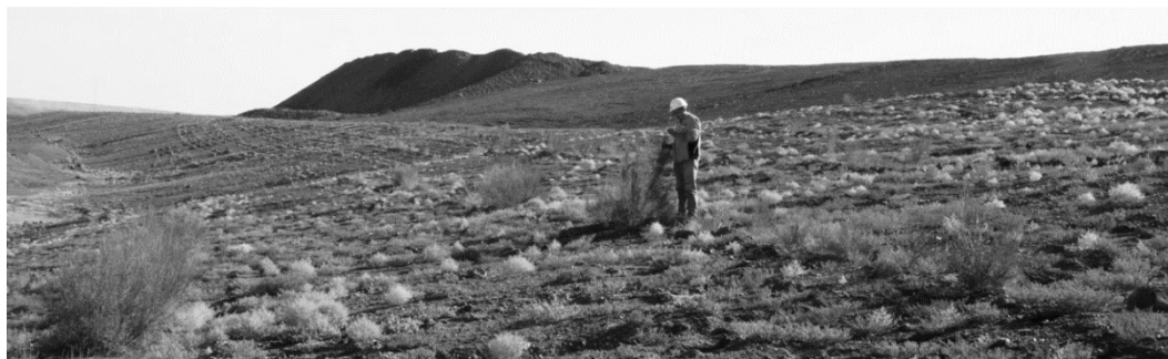
Figure 1 Rehabilitation work conducted at Sunset pit
