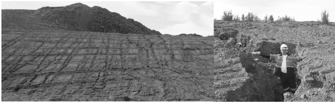
Figure 9 Cracks occurred due to flood of heavy rain at rehabilitated area
