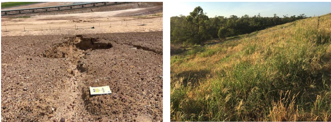
Figure 5 Left: Gully and tunnel erosion on Moranbah North spoil pile pre-treatment March 2016. Right: Stabilised mound with well-established body of grass post-treatment (March 2017)
