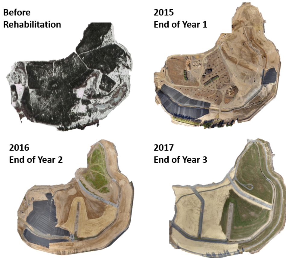
Figure 2 Aerial imagery showing the advancement of the TMA-2 rehabilitation work
