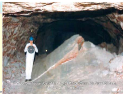
Figure 6 Massive floor strata uplift
