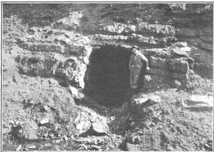
K. TUNNEL OPENING IN WHALERS CREEK COAL SEAM.
