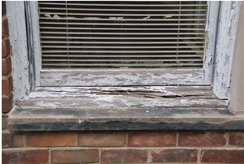
WINDOW #17 SPLIT SILL / BOTTOM SASH RAIL
