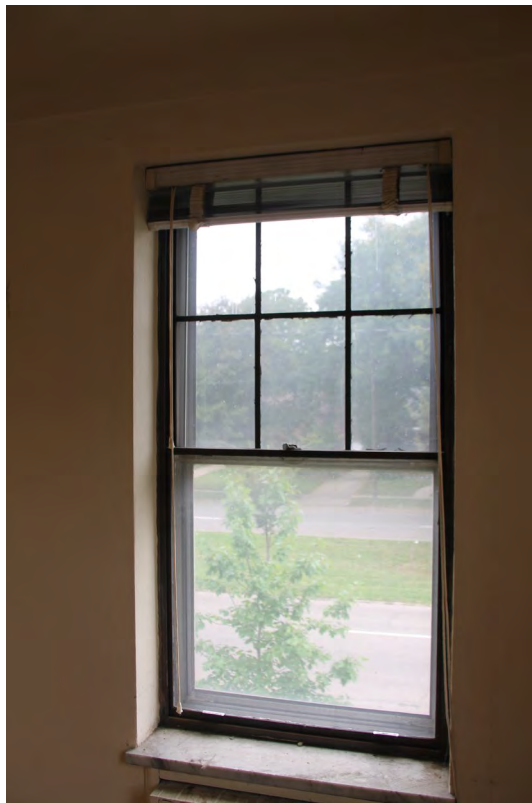
WINDOW # U19 INTERIOR VIEW
