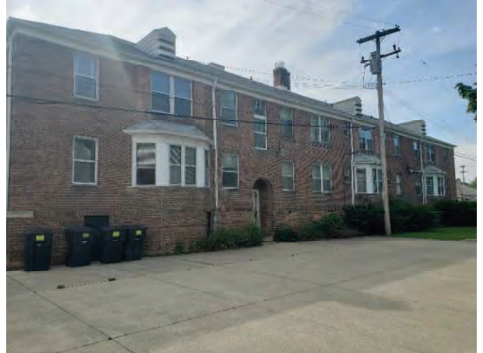
Fig-17 9710 rear (west) façade
