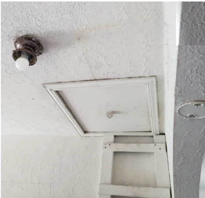
Fig-27 Attic access
