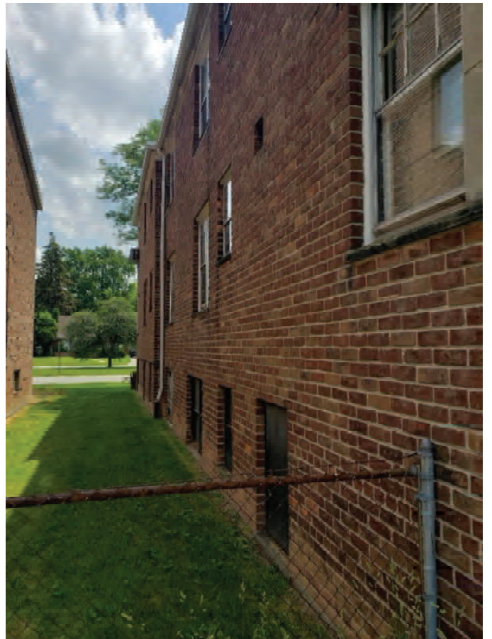
Fig-4 North facade
