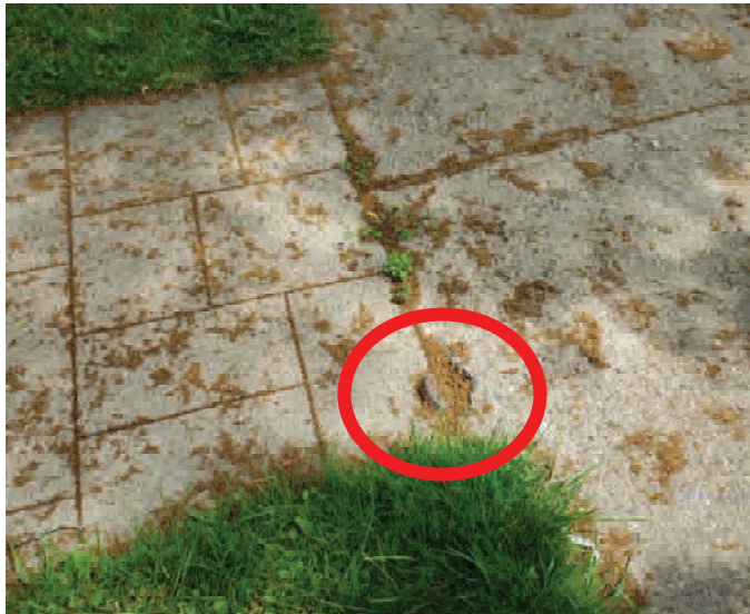
Fig-14 Utility cap in sidewalk
