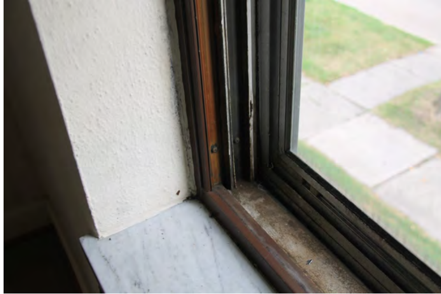
WINDOW #U19 INTERIOR JAMB TRACK TYPICAL
