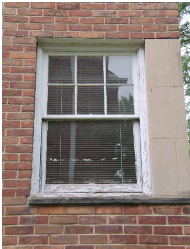
WINDOW #17 FULL VIEW/ EXTERIOR
