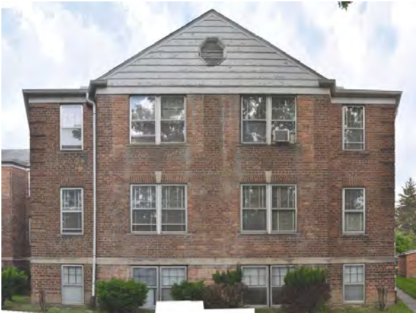
East Elevation - Southern Facade
