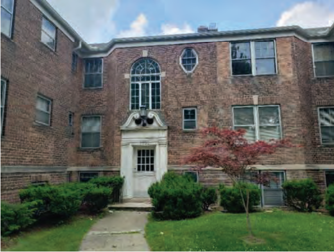
Fig-15 9730 front (east) façade
