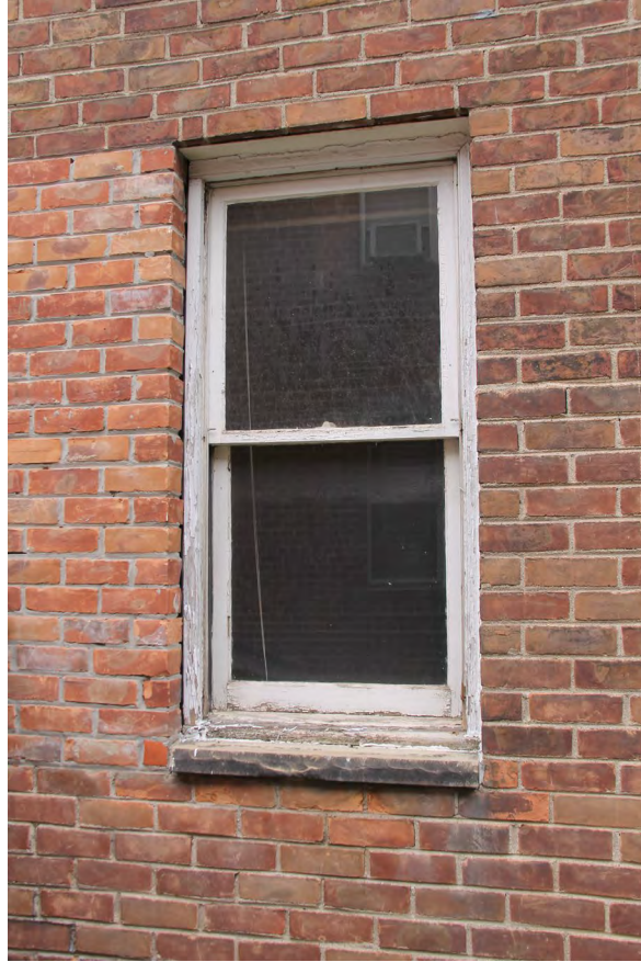
WINDOW #H3 FULL VIEW / EXTERIOR
