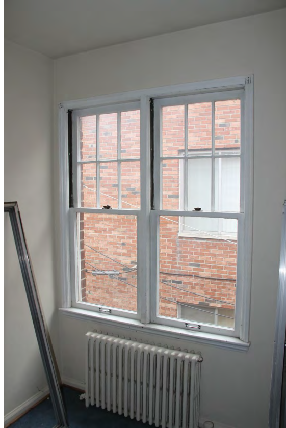
WINDOW #H4 INTERIOR SILL AND MULLION
