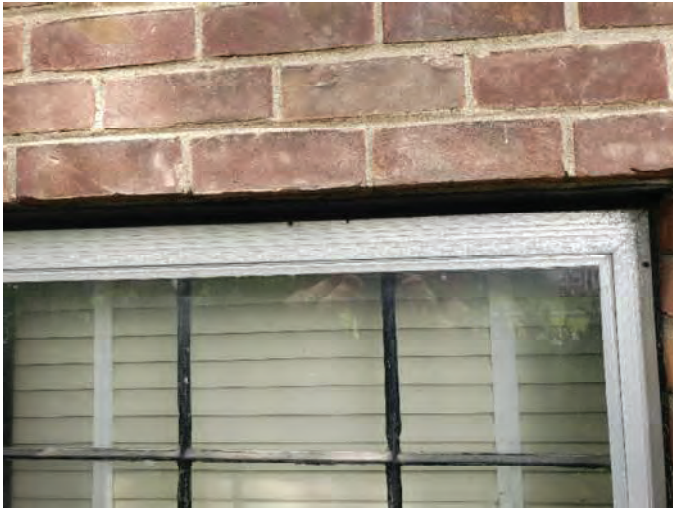
Fig-5 Typical lintel condition
