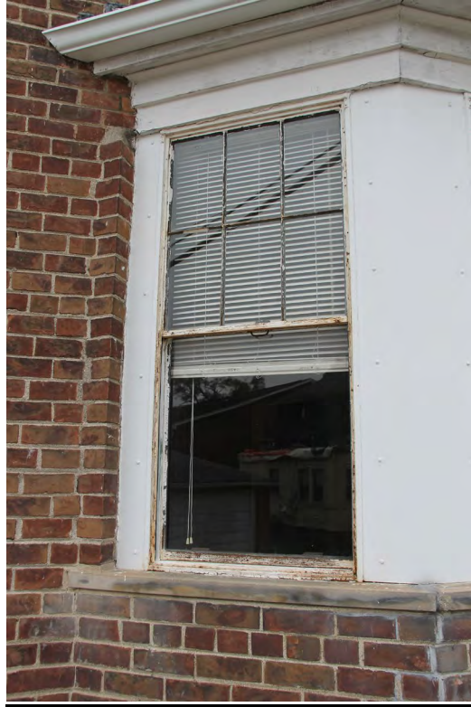
WINDOW #W2 EXTERIOR VIEW
