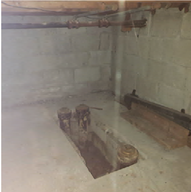
Fig-10 Sump pit
