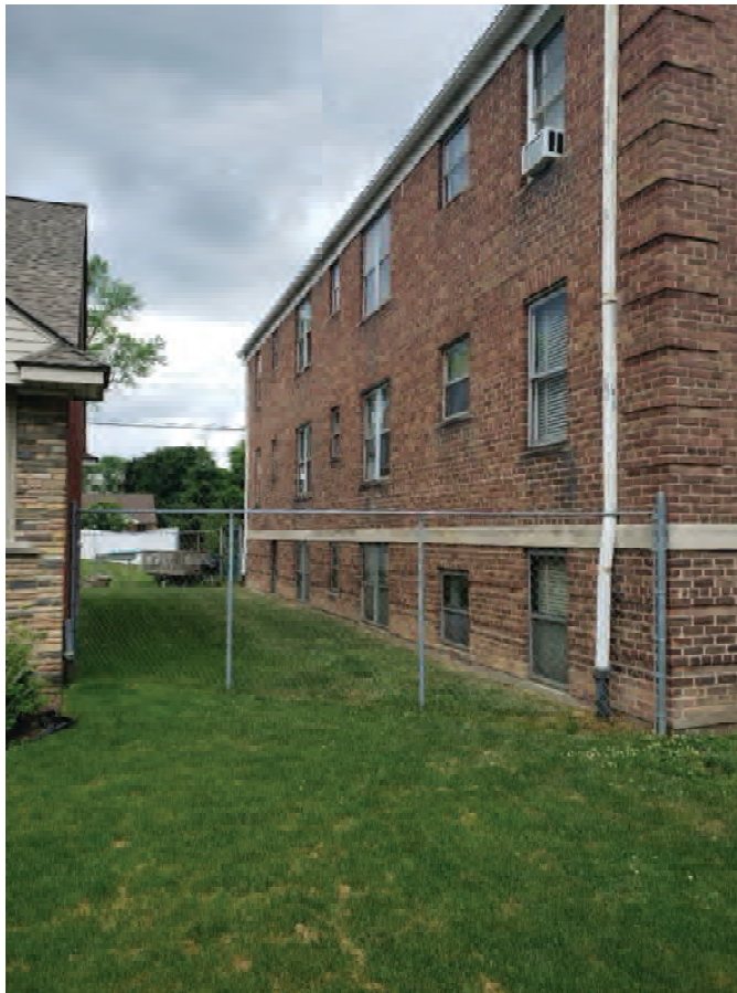
Fig-16 9710 south façade
