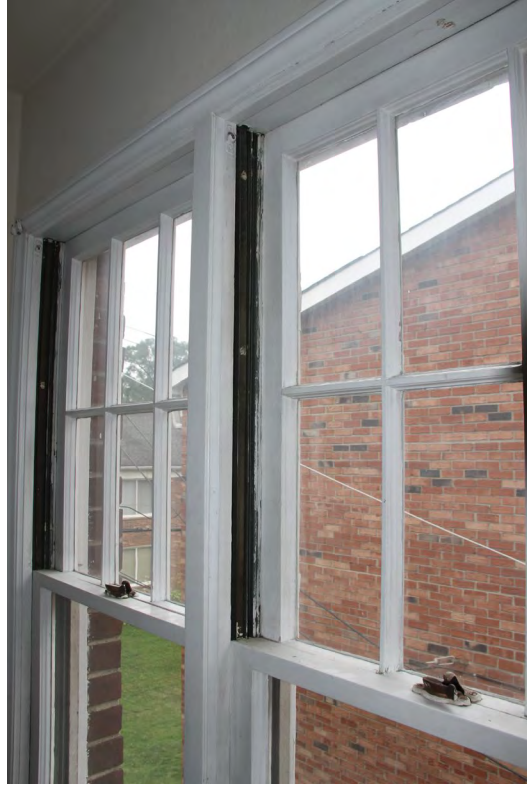
WINDOW #H4 INTERIOR VIEW INTERIOR MULLION
