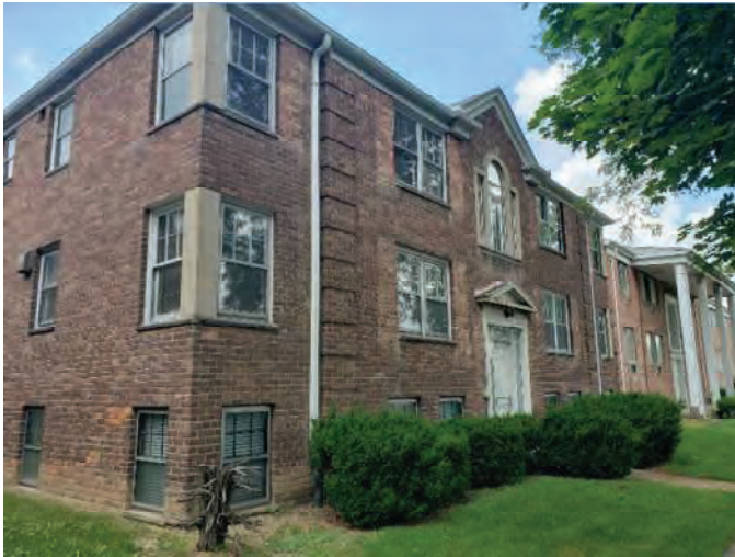
Fig-1 9710 Front (east) façade
