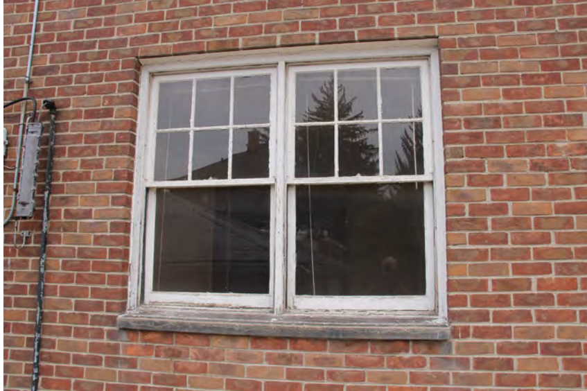
WINDOW #E3 FULL VIEW / EXTERIOR
