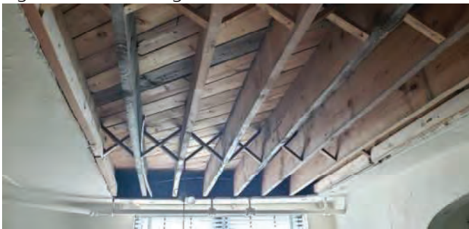
Fig-31 Typical joist condition at exposed ceilings
