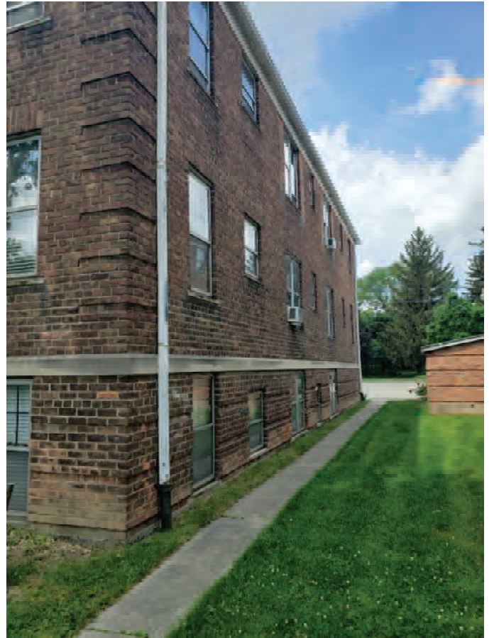
Fig-18 north facade
