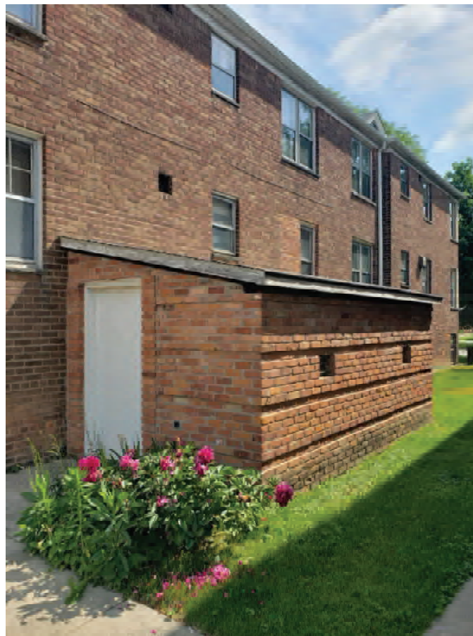
Fig-2 9710 South façade
