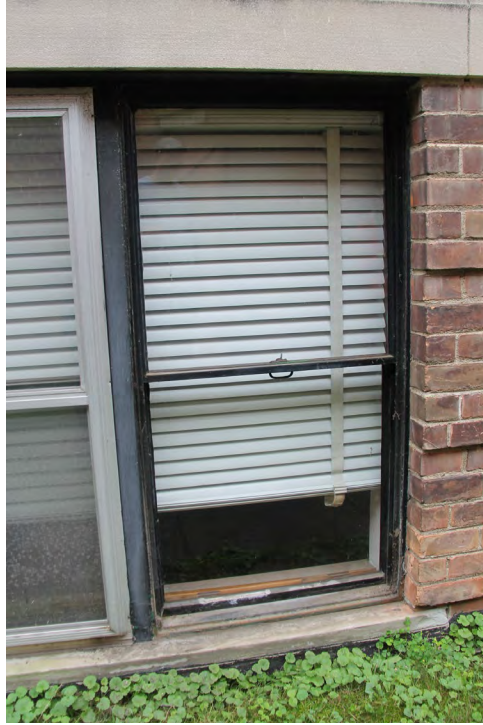
WINDOW #P5 EXTERIOR VIEW
