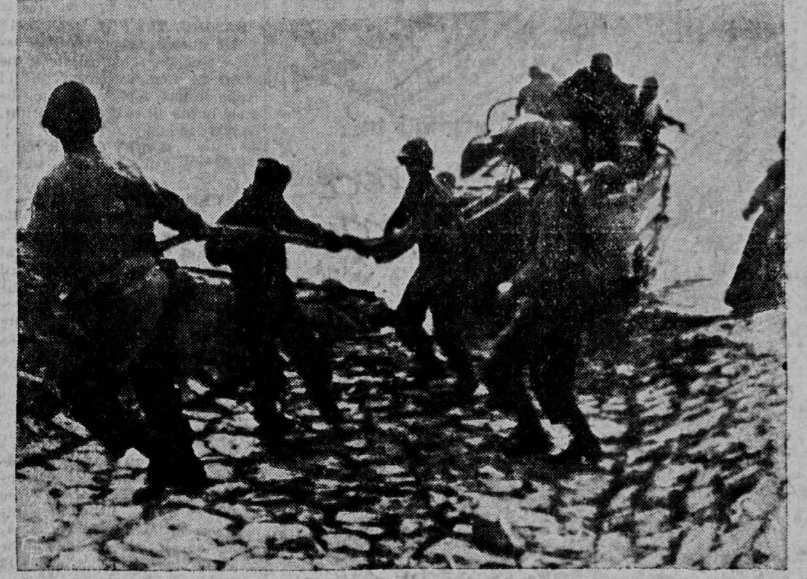
SHOWN ON THE BANK OF THE GREAT Rhine river in Germany are signal corpsmen of the United States Ninth army who are stringing submarine communications cable across the watery barrier, as they endeavor to keep the communications service up with the fast-advancing troops breaking out into the heart of Germany's Ruhr area. This is a United States army signal corps radiophoto.
