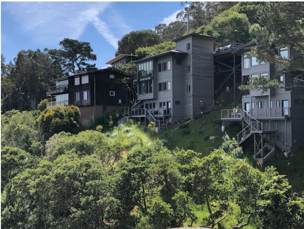
Fig.2 – 48-50 Marion Ave. (left), 60 Marion Ave. (center), 62 Marion Ave. (right) looking south from north end of Marion Ave.
