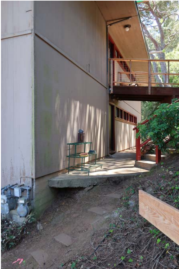
Fig.9 – 40-42 Marion Ave., front (west), looking south
