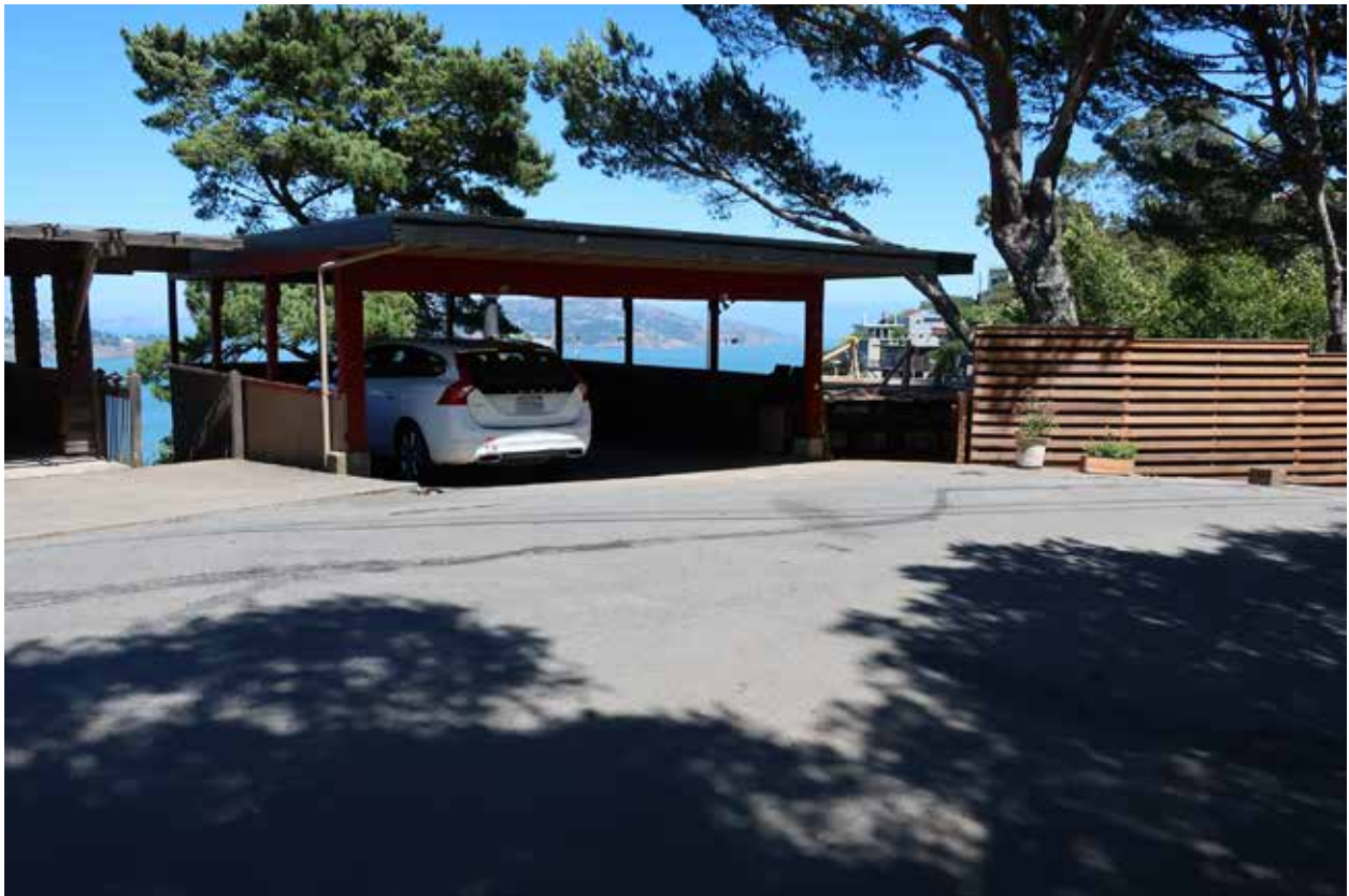
Fig.2 – 40-42 Marion Ave., carport and front fence from street (looking east)
