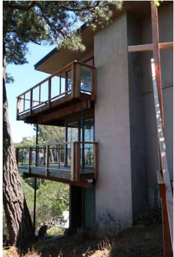
Fig.6 – 40-42 Marion Ave., north side
