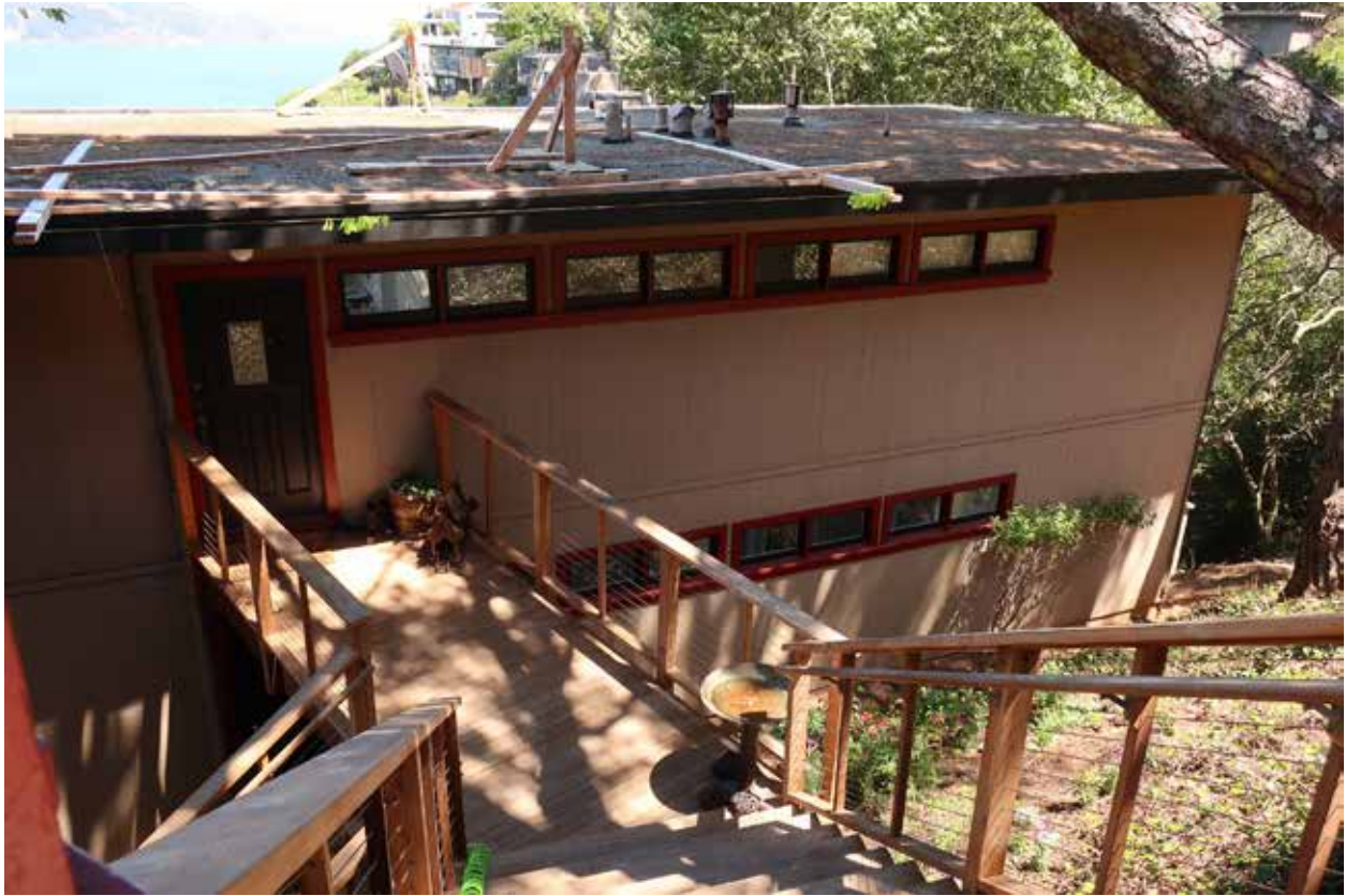
Fig.3 – 40-42 Marion Ave., front (west) from top of entry stairs (looking east)
