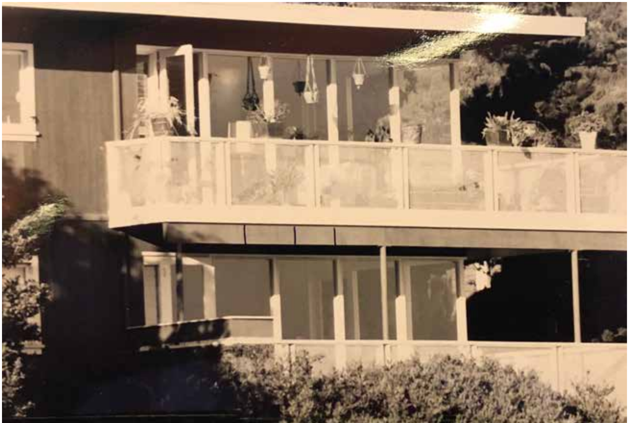
Fig.10 – 40-42 Marion Ave., part rear view (from 1976 permit application)
