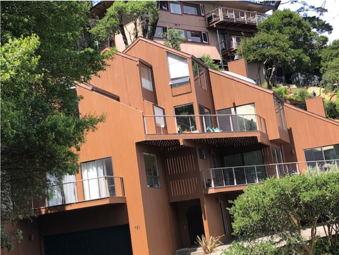
Fig.6 – 101-103 Edwards Avenue with 40-42 Marion Ave. above, looking from Edwards Ave.
