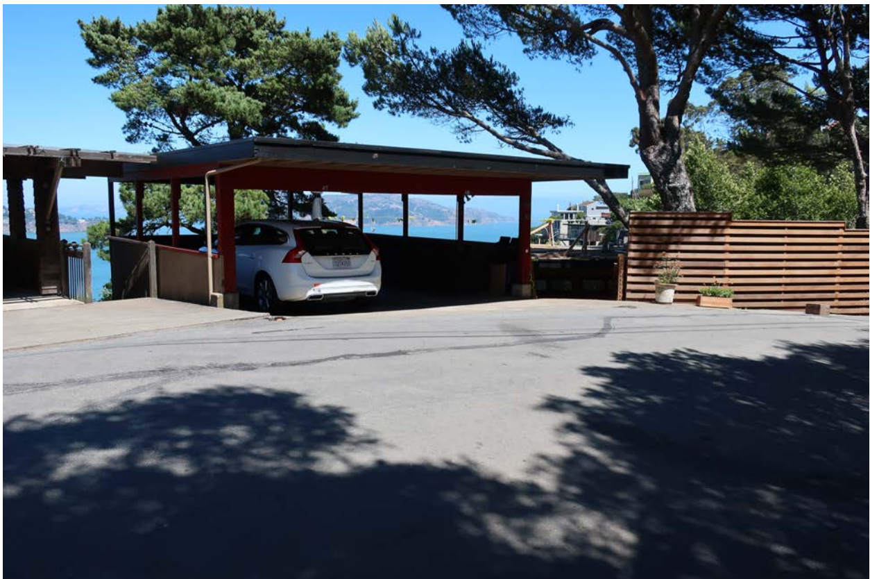
Fig.6 – 40-42 Marion Ave., carport and front fence from street (looking east)
