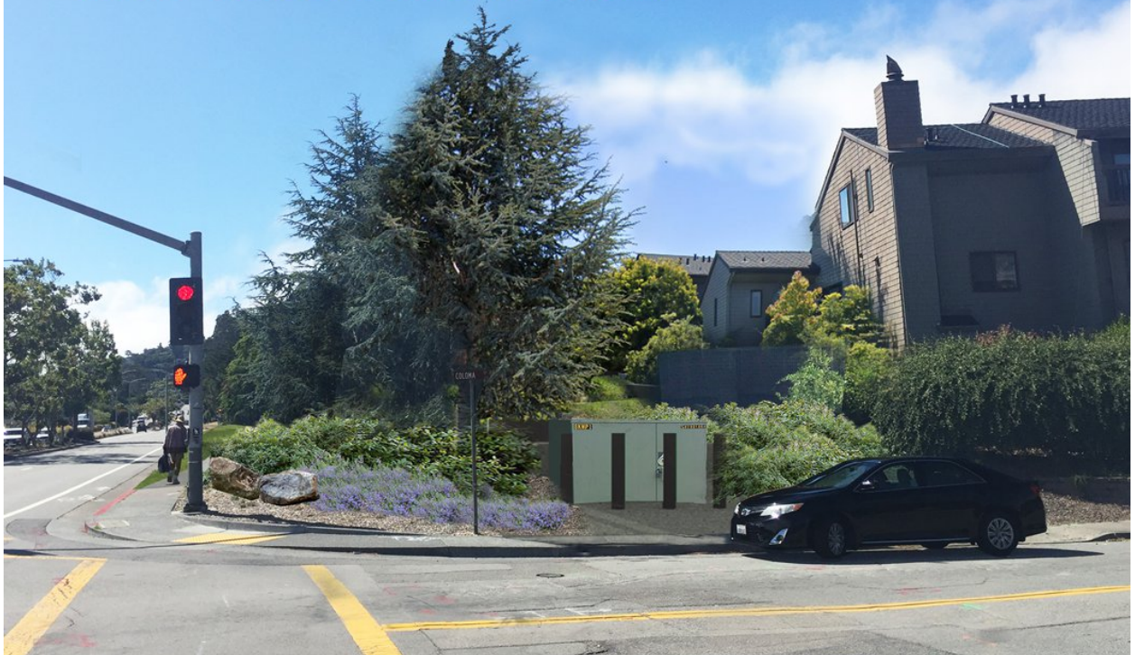
VIEW 2 YEARS AFTER CONSTRUCTION
