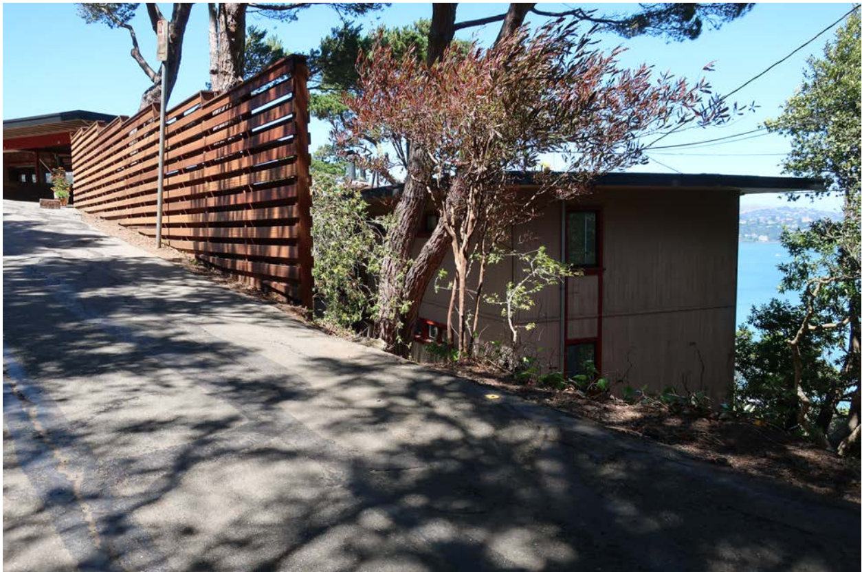
Fig.5 – 40-42 Marion Ave., south side and front fence from street (2018, looking north)
