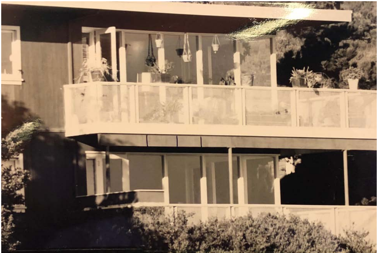
Fig.14 – 40-42 Marion Ave., part rear view (from 1976 permit application)
