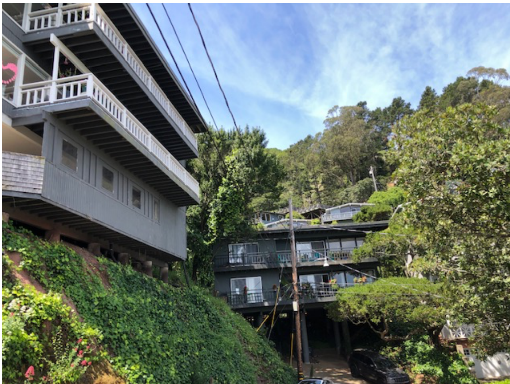
Fig.8 – 121-123 Edwards Ave. (left), 127-129 Edwards Ave. (center) looking from Edwards Ave.
