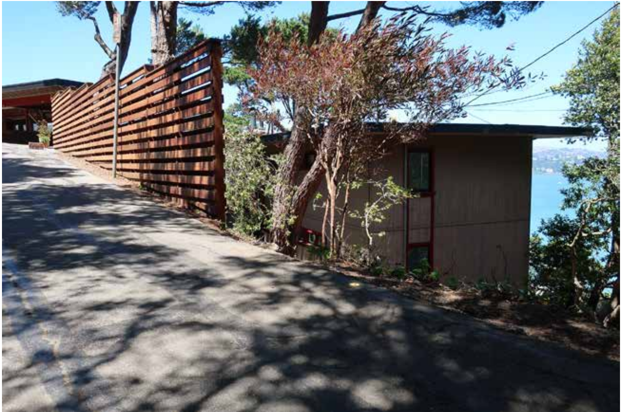
Fig.1 – 40-42 Marion Ave., south side and front fence from street (looking north)
