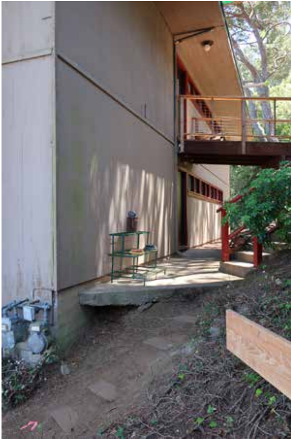
Fig.5 – 40-42 Marion Ave., front (west), looking south
