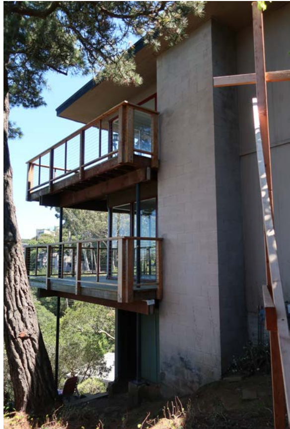
Fig.10 – 40-42 Marion Ave., north side
