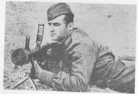
CZECH RECOILLESS ANTITANK GRENADE LAUNCHER P-27 "PANCEROVKA."
