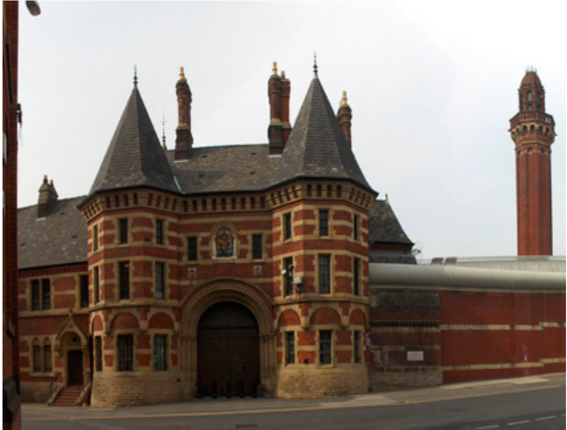
Fig 4.5 The gatehouse at Strangeways, with the cooling tower in the background (HeatherBurnside.com)
