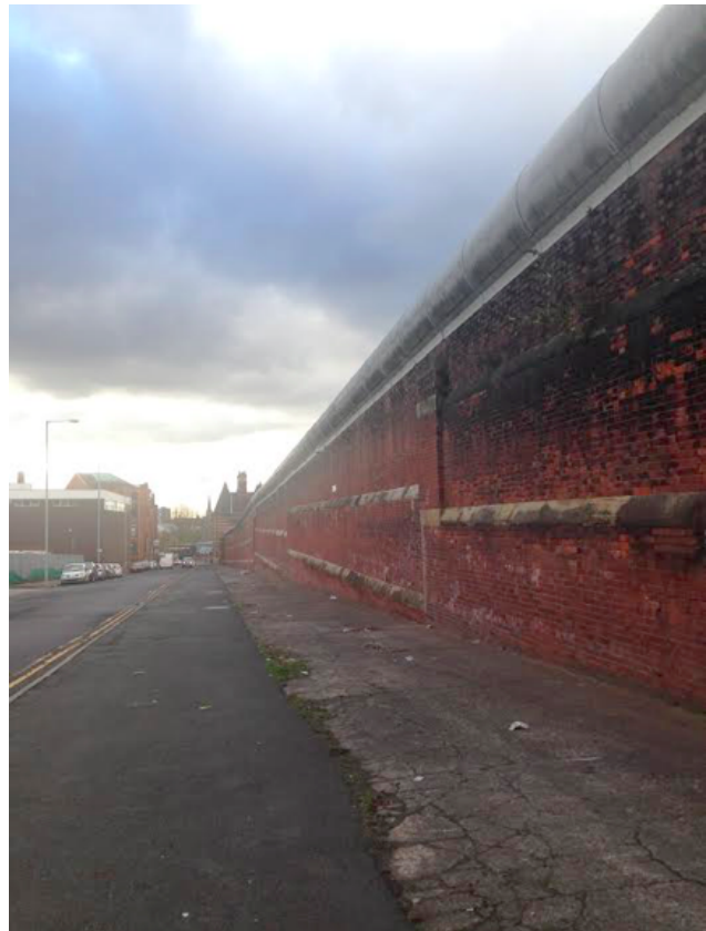
Figs 7.8 (left), 7.9 (right) Two further images of Strangeways' walls taken by Carl. Fig 7.8 shows the wall as it has been reconstructed since the 1990 riots, whereas Fig 7.9 shows one of the remaining sections of original 1860s wall.
