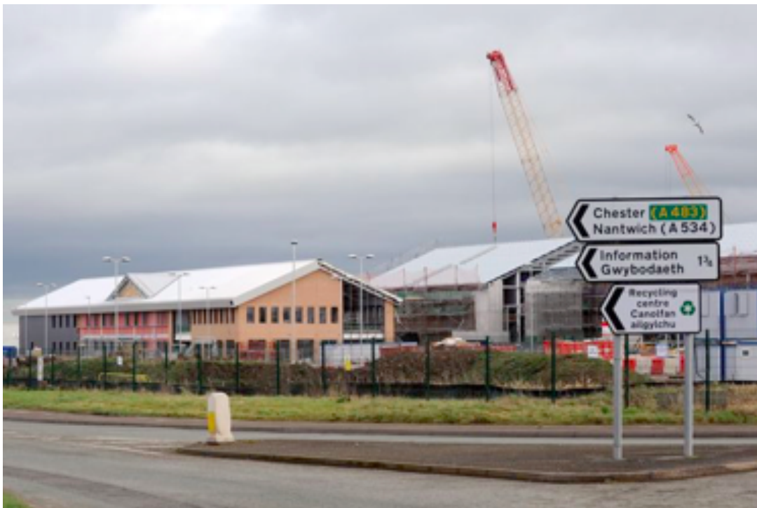
Fig 8.4 Berwyn under construction, 2016.
