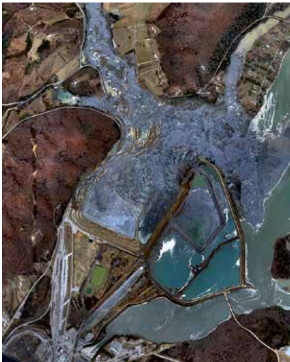
Fig 13. The aerial image of the Tennessee fly ash spill area acquired soon after the spill. (Image courtesy of Tennessee Valley Authority and can be viewed at http://www.tva.gov/kingston/photo_gallery/pages/123002.htm )
