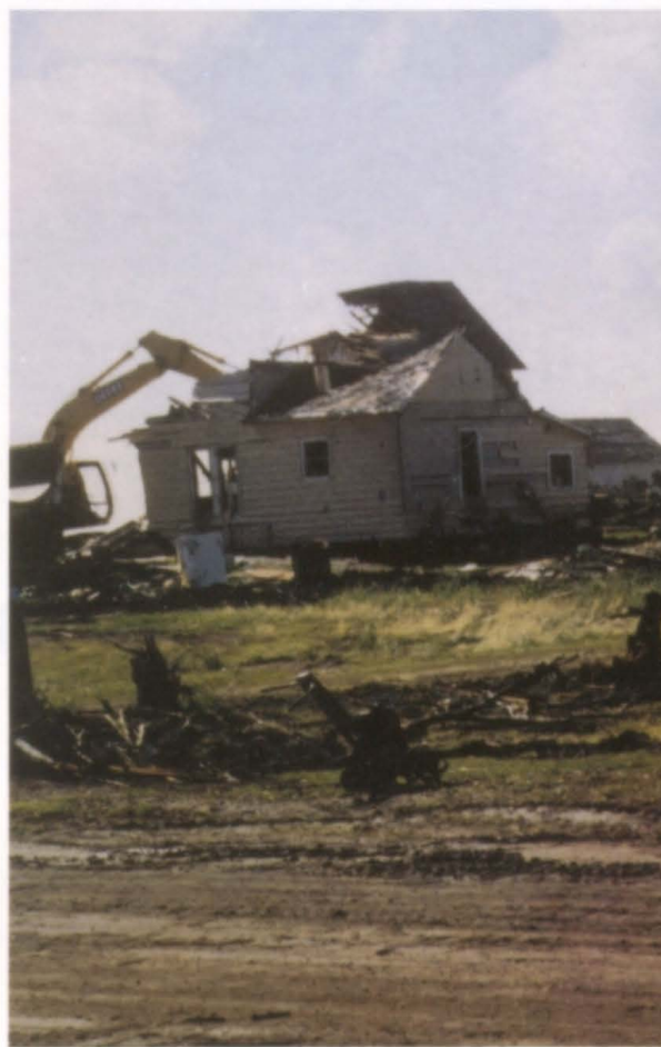
Bulldozing memories. A damaged home is torn down.
