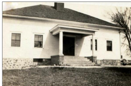
The "new" District No. 4 school building. Photos from the Town of Pavilion's collection.
