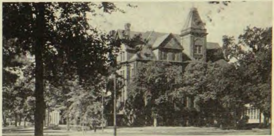
The Building Which Houses the School of Business
