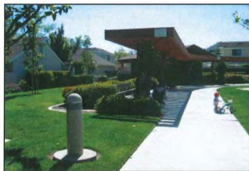
3.2.2.1 f) Multi-family development is enhanced with the inclusion of pedestrian paths and transit connections.
