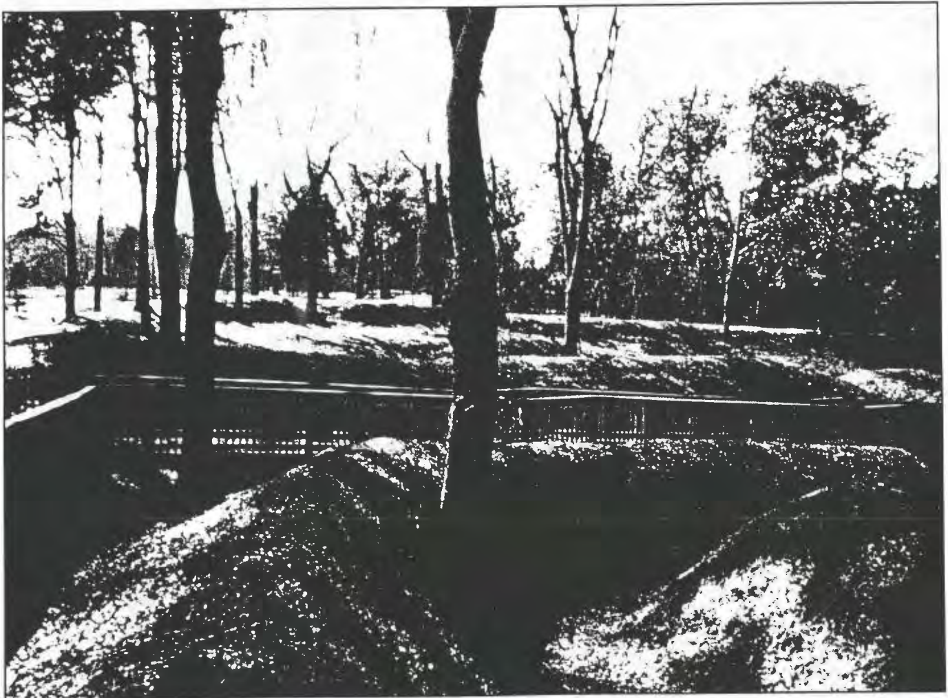
To provide access to the historic earthworks at the Stones River National Battlefield in Murfreesboro, Tennessee, an interpretive boardwalk was installed [preceding page and above] to allow visitors access to the resources while protecting the earthworks themselves. (courtesy NPS)
