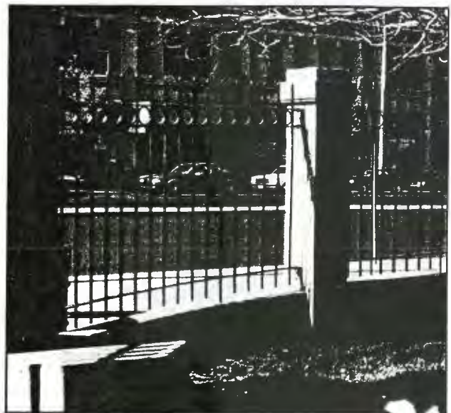
A section of the wall surrounding the Dorchester North Burying Ground in Massachusetts was in a state of advanced deterioration. [top] than reconstruct the failing wall along the main entrance area, only its piers were replaced. [bottom left] The area of wall between these pi replaced with an iron fence. [bottom right] This approach was selected to improve the perceived safety and security of the burial grou allowing for visual access into the burial ground, where it was previously enclosed. (author, 1993 and Boston Parks)
