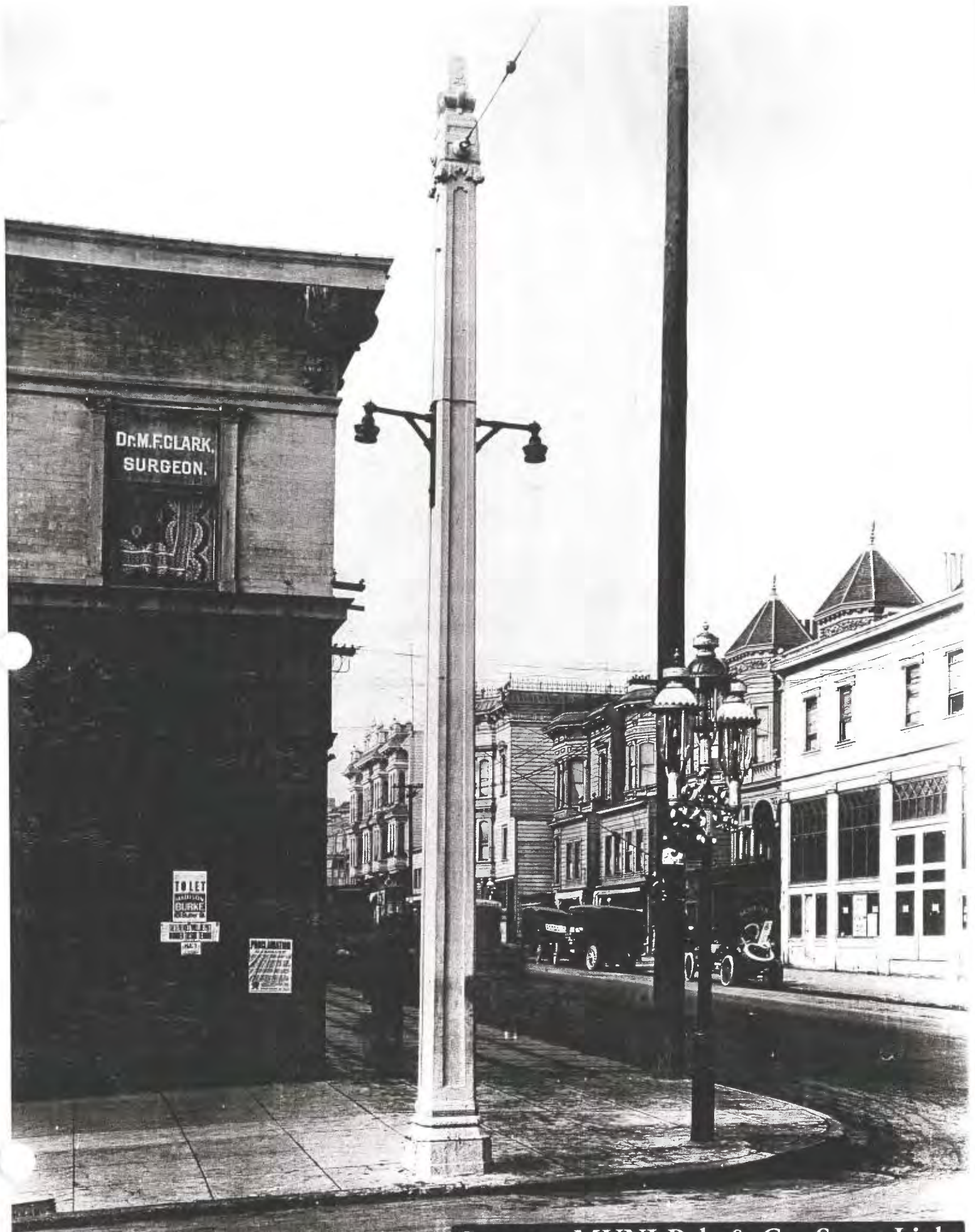
Concrete MUNI Pole & Gas Street Light
