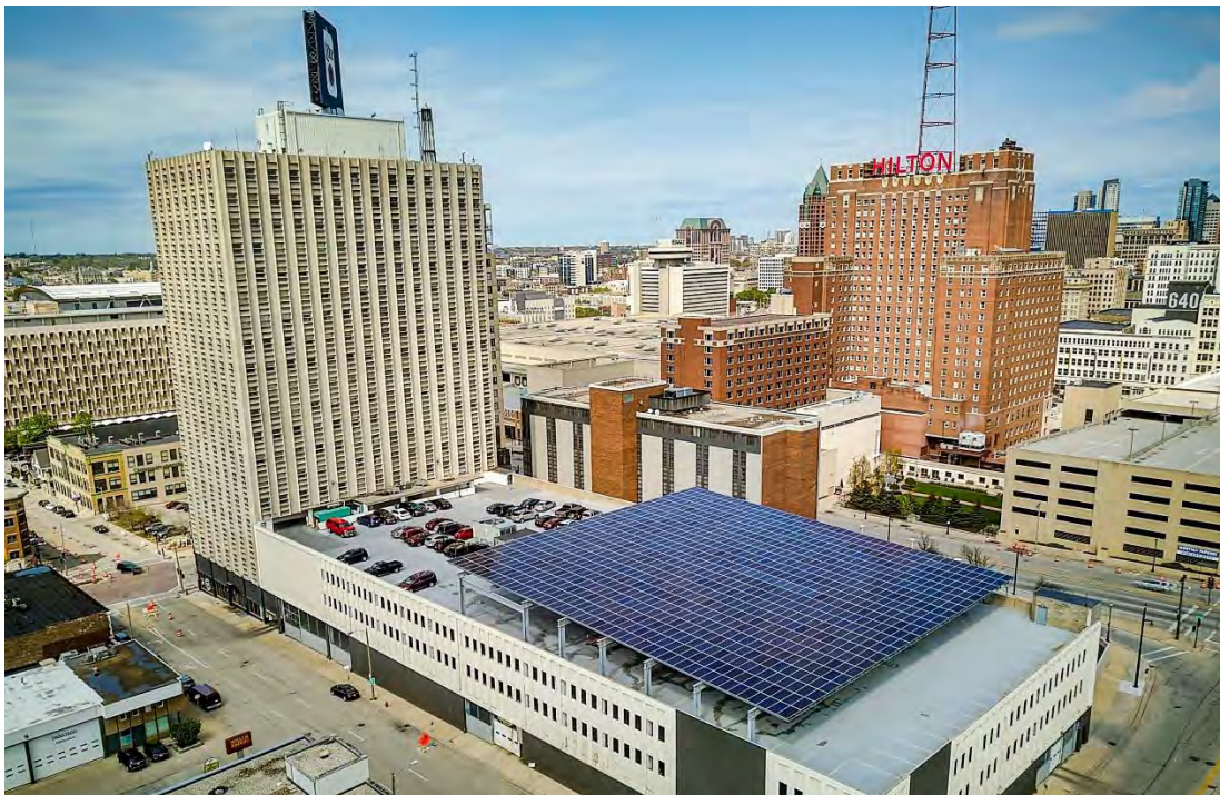
Clark Building Solar Canopy
