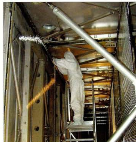
Wiring and photomultiplier mounting for the T600 ICARUS prototype.
