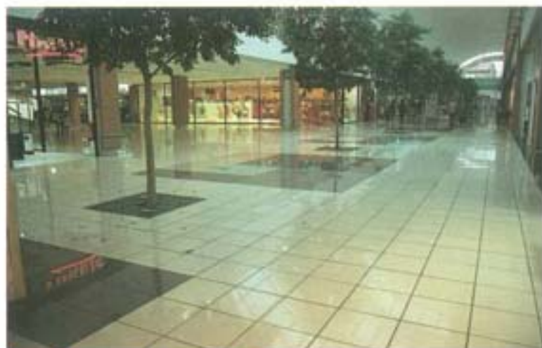
Cora Shopping Center in Chatelaineau Remodeled floor: 3,500 m 2 (37,600 sq. ft.)
