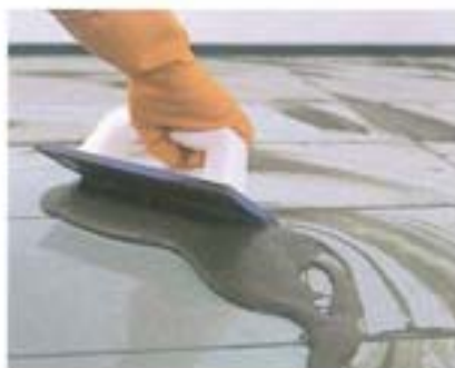
Grouting with MAPEFONIC GROUT
