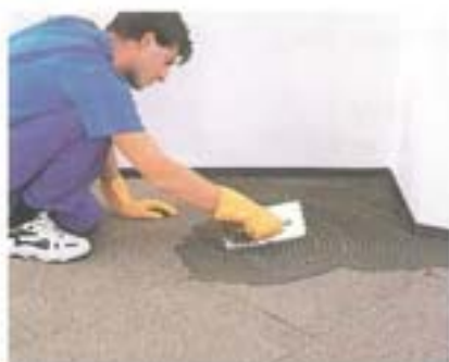
Spreading MAPEFONIC MORTAR on MAPEFONIC PAD
