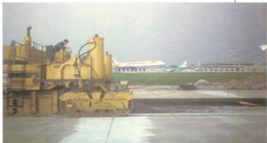
Using MAPEFLUID X404: Marco Polo Airport, Venice, Italy
