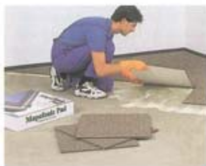
Applying MAPEFONIC PAD over MAPEFONIC GLUE
