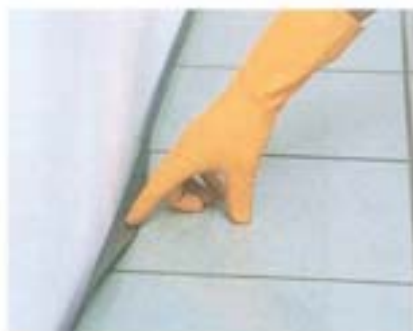
Installing baseboards: fold the MAPEFONIC STRIP back up over the edge of the surface of the flooring. Remove the excess MAPEFONIC STRIP with a cutter
