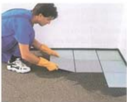
Laying ceramic tiles over MAPEFONIC MORTAR
