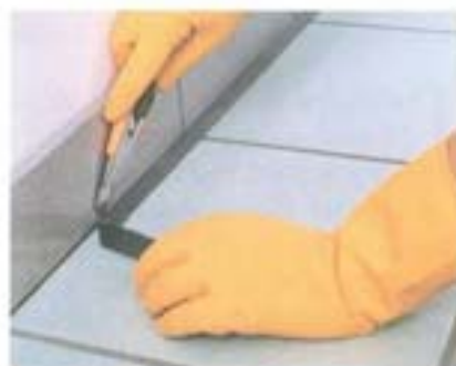
Installing baseboards: fold the MAPEFONIC STRIP back up over the edge of the surface of the flooring. Remove the excess MAPEFONIC STRIP with a cutter
