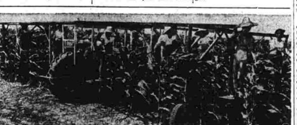
Twelve Girls on a Rig: This machine was invented by Lester Pfister to speed delasseling the 4523 acres of seed corn he plants each year. Rig moves at speed of one-half mile per hour. De-tasseling
