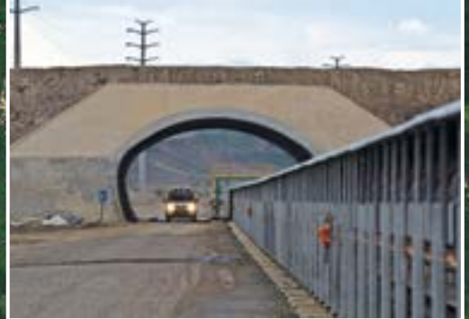
Sapta Bridge, where the conveyor passes under a mine road.
