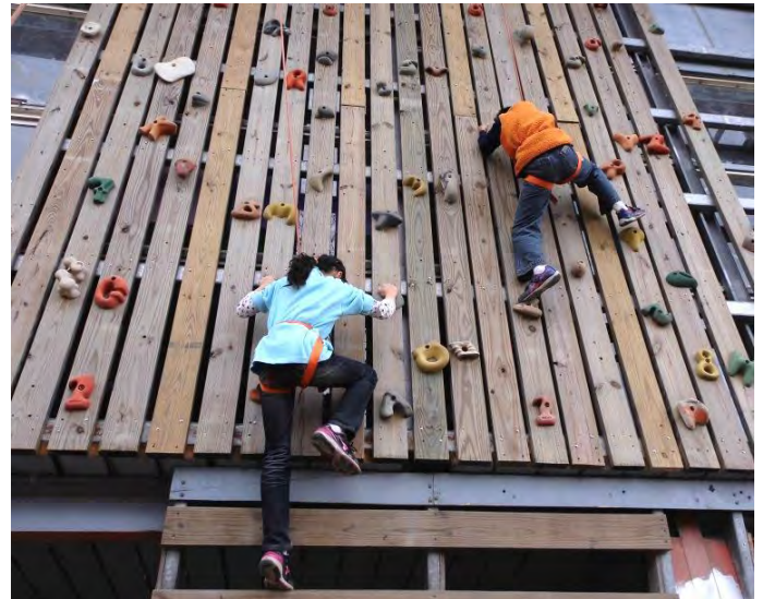
Climbing Wall - It is a side wall of Tian-Ren Climbing House
