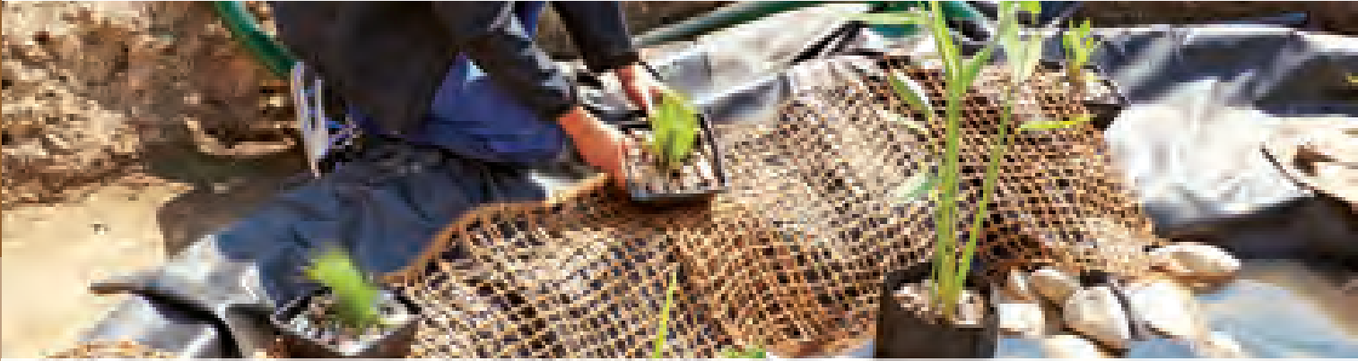
Application example: Embankment mat
