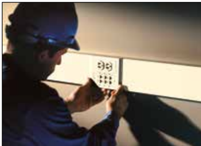
Prewired Raceway gets installers off the job in 1/3 less time than conventional raceway installations.
