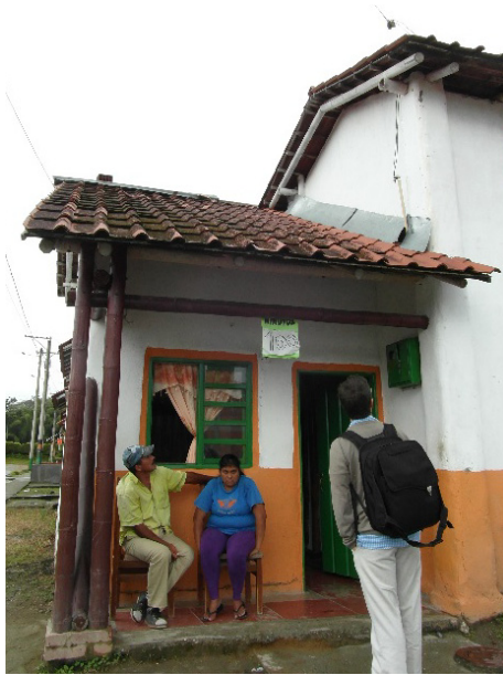
Figure 22: Post-earthquake engineered bahareque housing in Barcelona, near Armenia (Kaminski, 2016)
