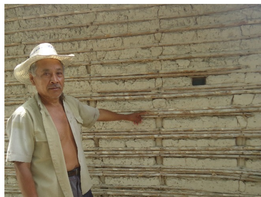
Figure 9: Caña brava (Costa Rica) or vara de castilla (El Salvador): Small diameter bamboo-like cane (Kaminski, 2016)
