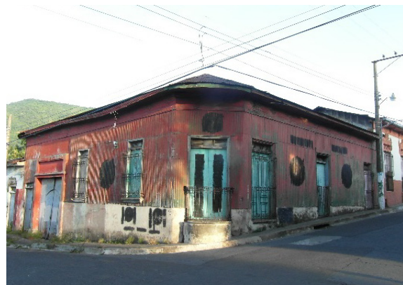
Figure 2: Traditional bahareque housing in Berlín, El Salvador. The outer render has been replaced with corrugated-iron sheeting (Kaminski, 2016)
