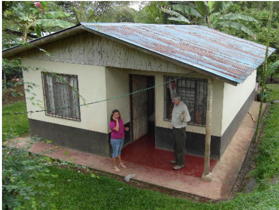
Figure 16: PNB house in Milano, Costa Rica – photo taken at 20+ years since construction (Kaminski, 2016)
