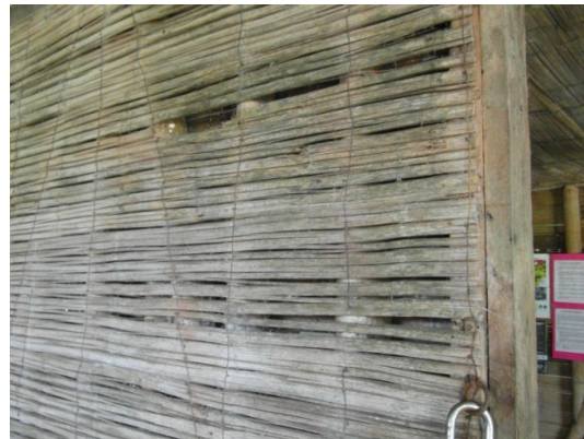
Figure 7: Esterilla (Colombia) or caña picada (Ecuador): Sheets of bamboo formed by physically opening / splitting a large diameter culm along its length and then unrolling it (Kaminski, 2016)
