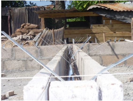
Figure 64: Photo of sole plate fixed to upstand with cast-in off-the-shelf steel straps, before casting straps into reinforced blockwork
