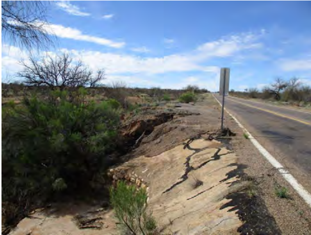
Figure 79: CMP inlet with concrete wing protection facing northeast
