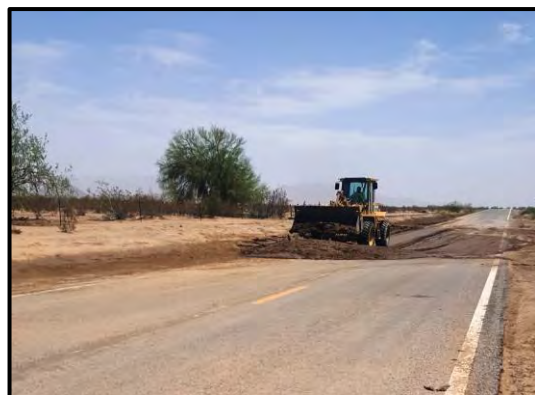
Figure 9. SR 238 at MP 25.67. Looking East
