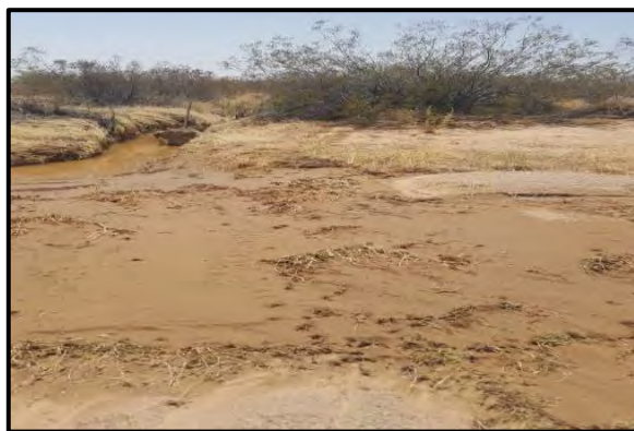
Figure 8. SR 238 at MP 25.25. Looking South
