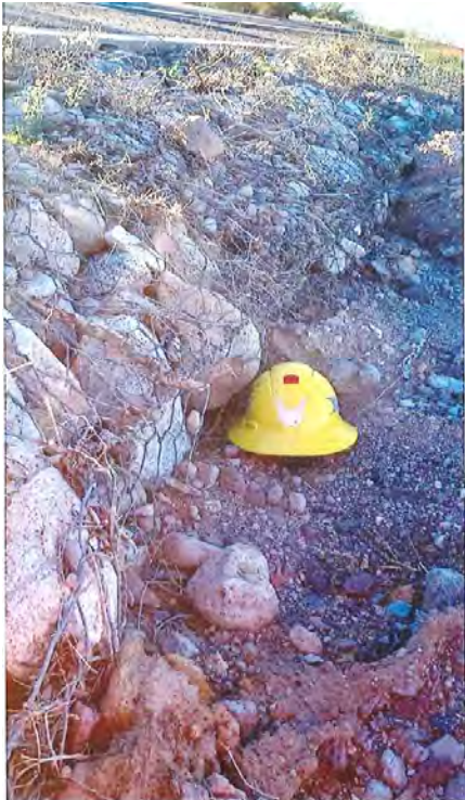
Figure 17: US 95 at MP 69.3
