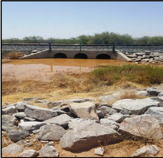
Figure 10. SR 238 at MP 31.83. Looking South
