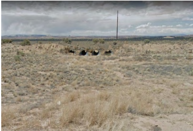
Figure 48: Northern View at Railroad Tracks (Picture Provided by ADOT)
