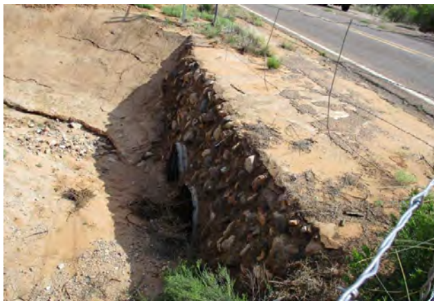
Figure 78: CMP outlet with concrete protection facing northwest
