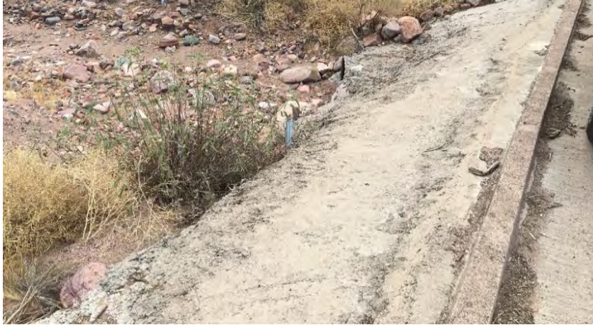
Figure 64: Southbound, Western View (MP 265)
