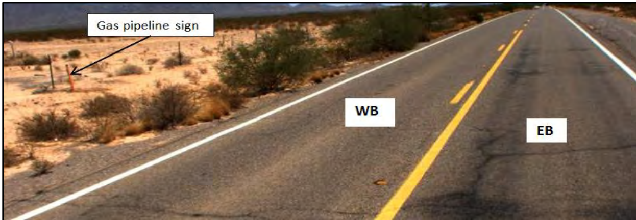
Figure 17. Existing Gas Pipeline crossing SR 238
