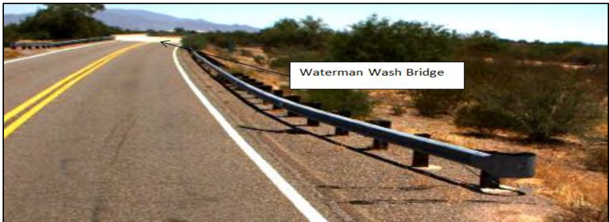
Figure 4. Existing Guardrail at the Waterman Wash Bridge
