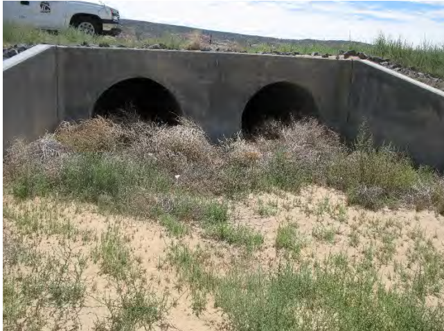
Figure 47: Pipe Culverts (Picture Provided by ADOT)
