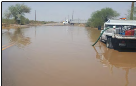
Figure 6. SR 238 at MP 31.80. Looking West
