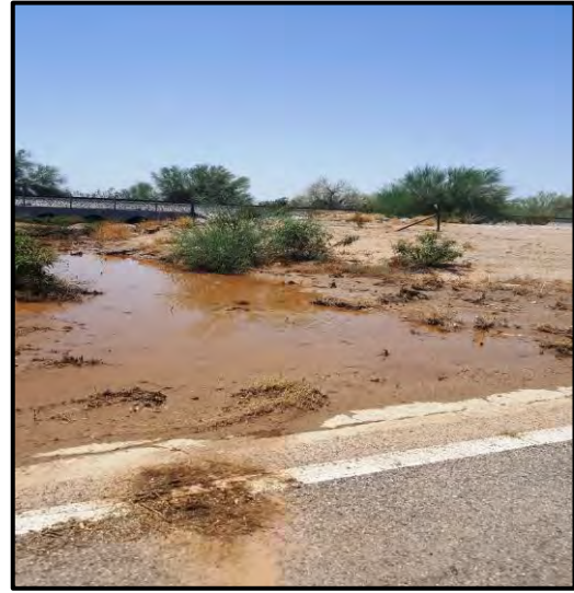
Figure 11. SR 238 at MP 26.32. Looking South
