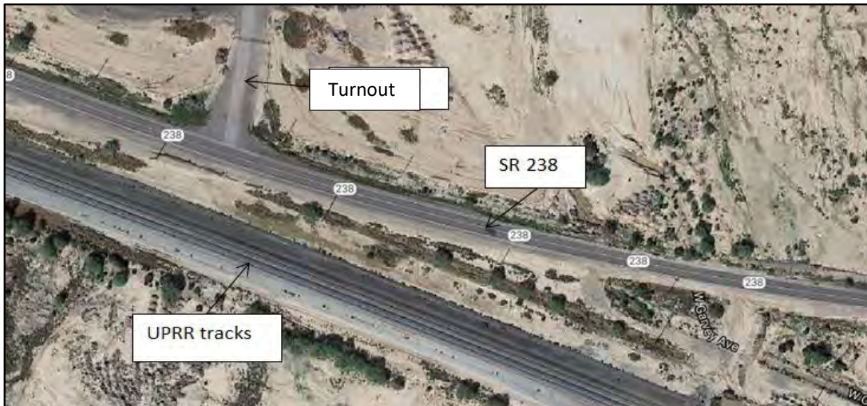
Figure 14. SR 238 & Railroad Tracks at MP 42.00
