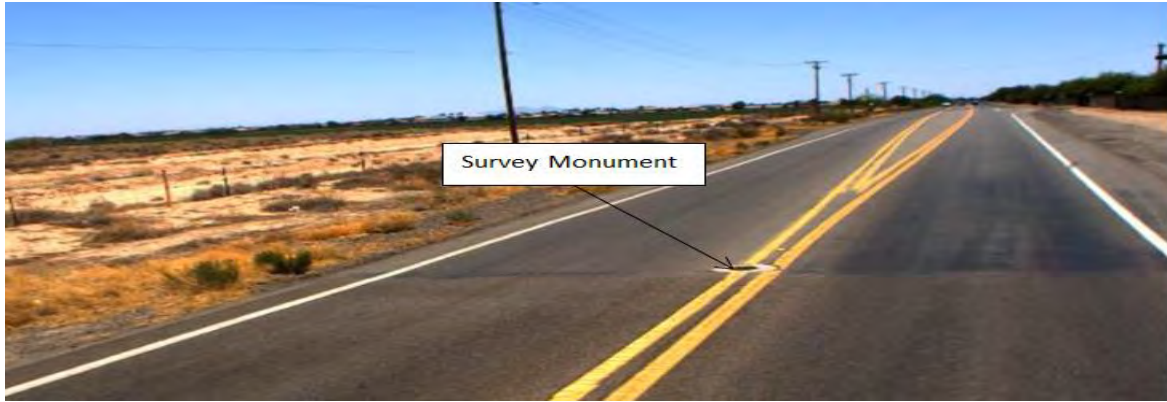
Figure 23. Existing Survey Monument at MP 43.55
