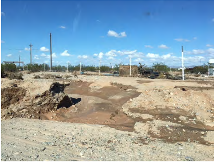
Figure 68: Sand Tank Wash near I-8
