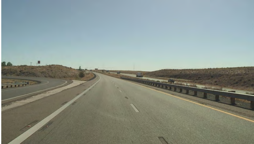
Figure 94: Westbound, Rear View (MP 287)
