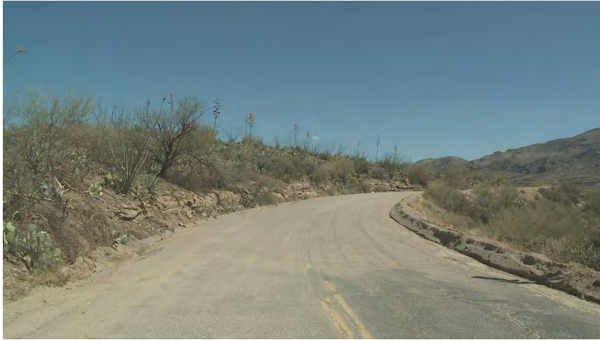
Figure 73: Westbound, Rear View (MP 220)
