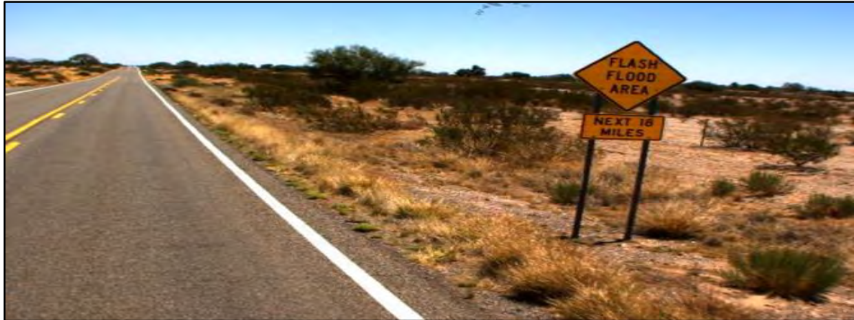
Figure 13. Flash Flood Area Sign at MP 25.02 (EB)
