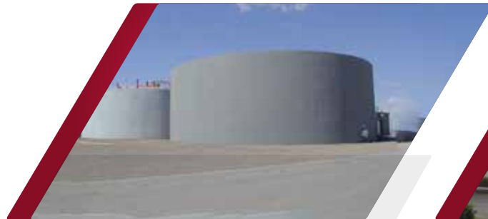
WATER/WASTE CONTAINMENT Treatment, Storage, Containment
