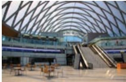
FIGURE 5. Top: ARTIC with radiant heating system installed, prior to the actual flooring being laid. Bottom: End result of the inside of ARTIC.
