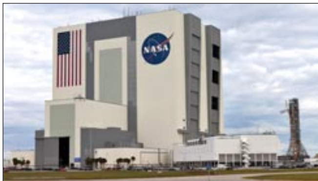
Seen to the right of the iconic Vehicle Assembly Building (VAB), a crane positions the Orion crew access arm (CAA) so it can be attached to the mobile launcher (ML). (NASA/Bill White)
