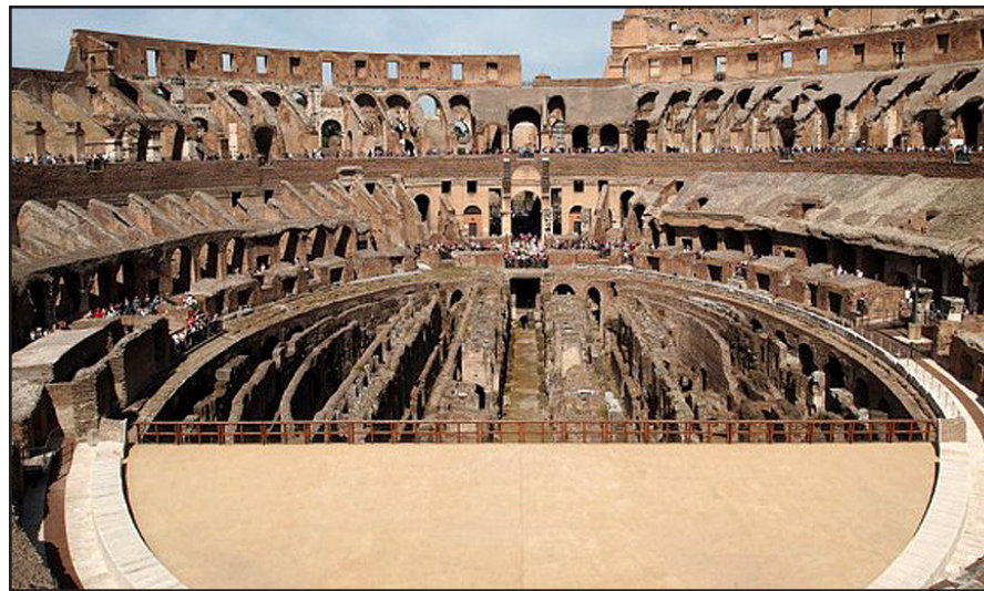
The partial reconstruction of the floor in the arena of the Colosseum.
