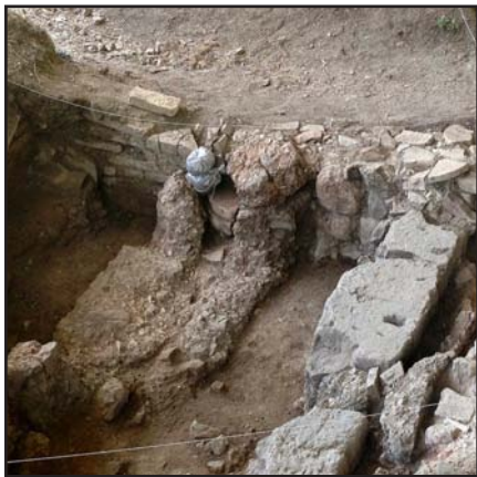
Fig. 3: (below) View of the chamber of Furnace 4 with its blocked opening.
