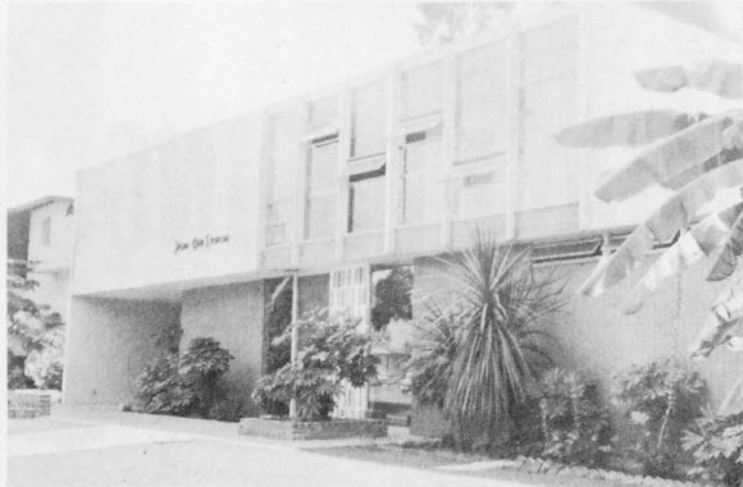
A beautiful, modern building was leased as the headquarters for the Los Angeles "Summer Invasion" program of Teen Challenge.
