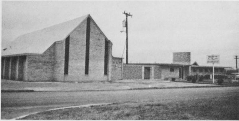
Previous Building Destroyed by Fire
