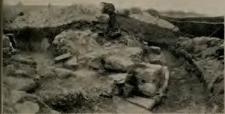
North East Corner of Fort.
