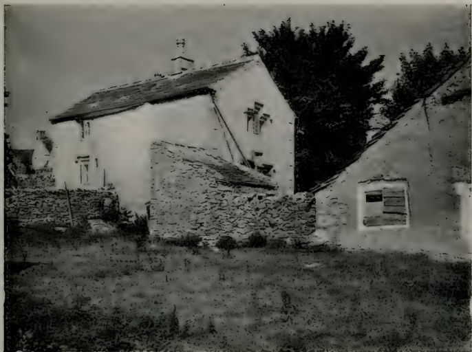
HOUSE AT LITTLE HUCKLOW (FROM THE SOUTH).
