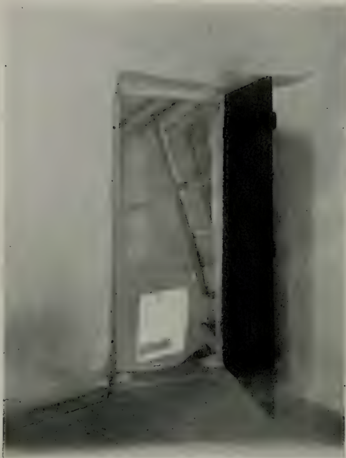
TOP OF STAIR IN UNDIVIDED HOUSE.
