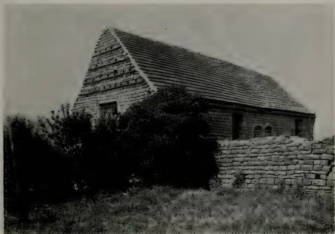
PADLEY HALL (FROM THE NORTH-EAST).
