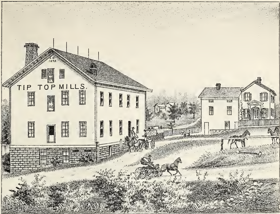
MILLS & RESIDENCE OF J. C. SCOTT & Co., NEW WATERFORD, COLUMBIANA CO., O.
