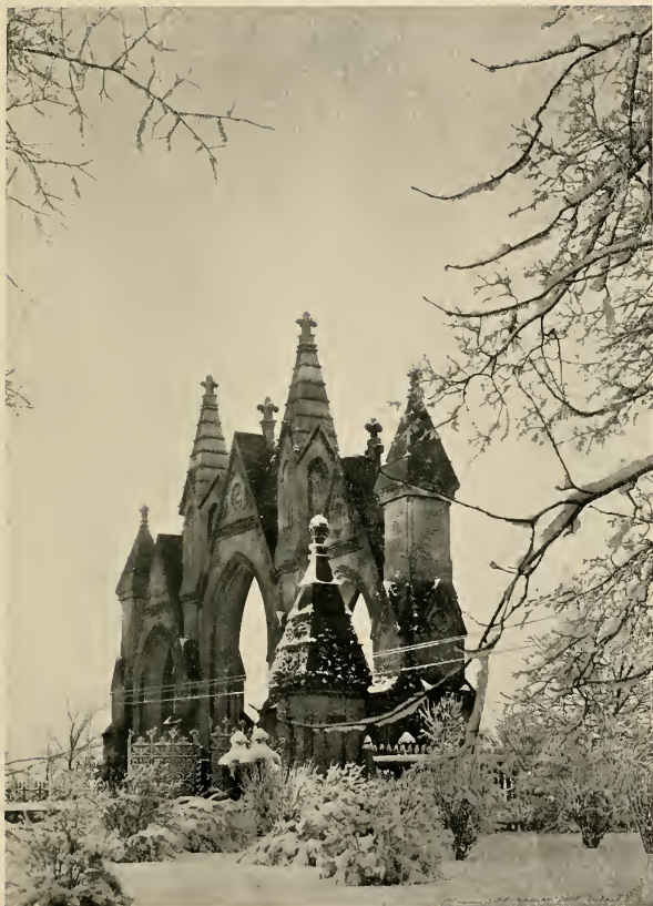
MAIN ENTRANCE—INSIDE VIEW
