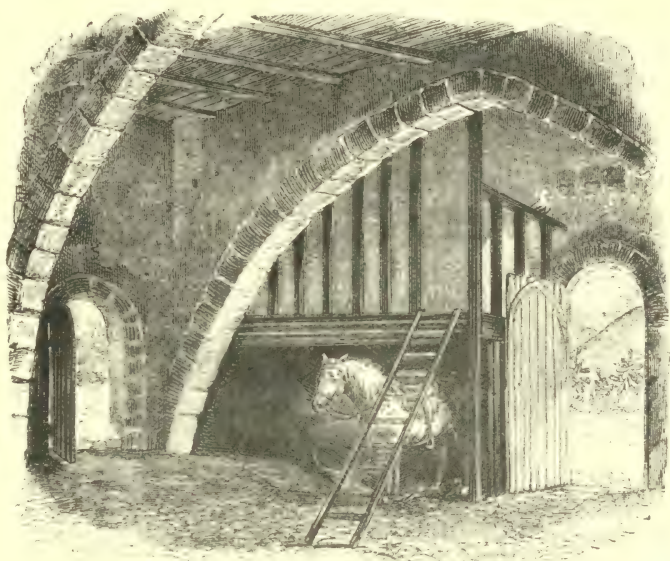
BUILDING USED AS A CHURCH AND SCHOOL. THE LOFT IS THE PASTOR'S STUDY.
