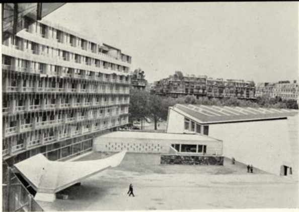
Secretariat façade, lobby and Conference Building. [Photo Unesco - D. Berretty]
