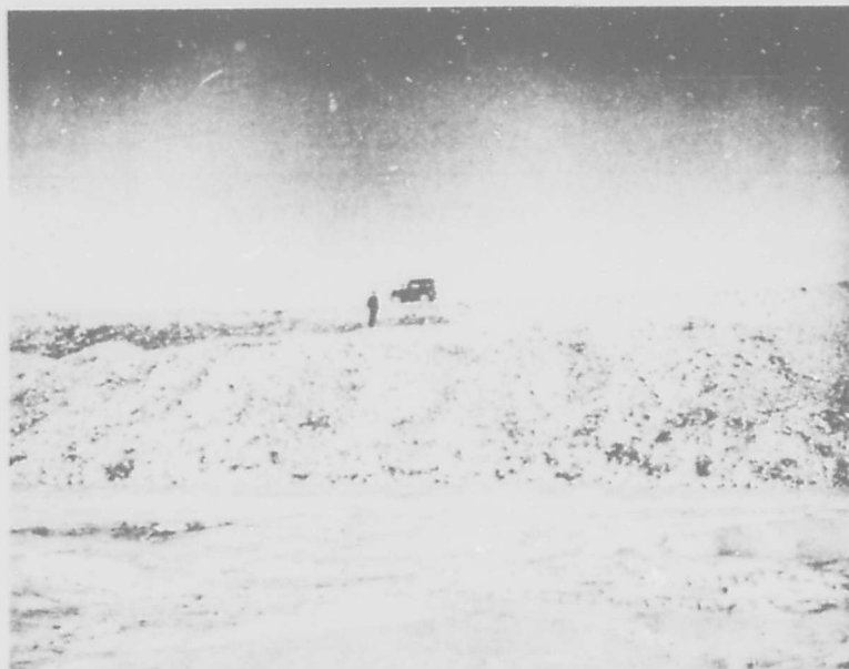
Figure 13. South side of Ramp Road, Station 4+00, 27 August 1959.
