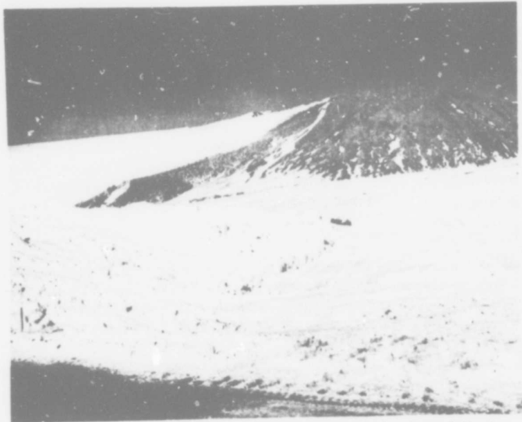
Figure 3. Snow removal along centerline of new Ice Tunnel Road. 5 June 1958.
