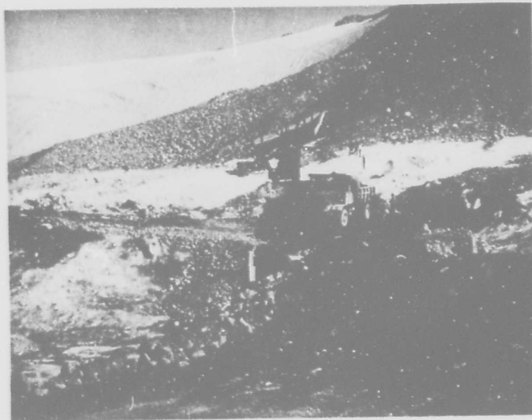
Figure 8. Cut section on new Ice Tunnel Road, 17 June 1958.
