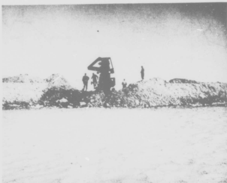
Figure 9. Ladder-type trenching machine cutting through ice ridge on Transverse Road, 24 June 1958.
