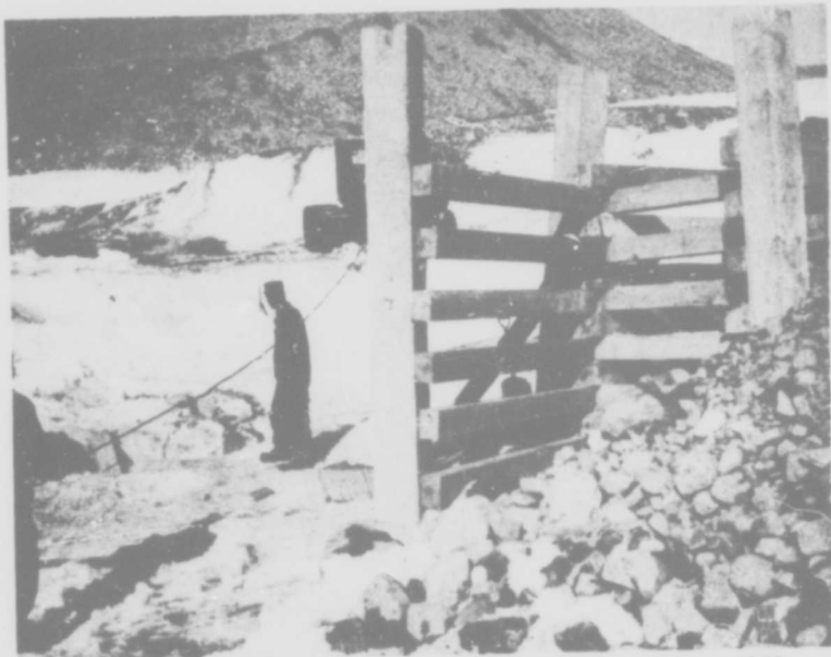
Figure 7. Construction of timber cribs on new bridge, 14 June 1958.
