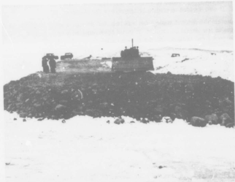
Figure 4. Fill being placed along new Ice Tunnel Road, 7 June 1958.
